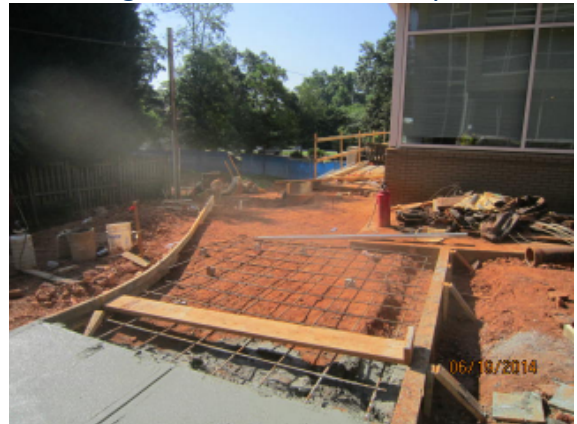
Pouring Sidewalk in Courtyard
