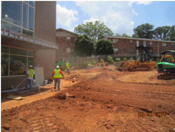
Grading for planter walls
