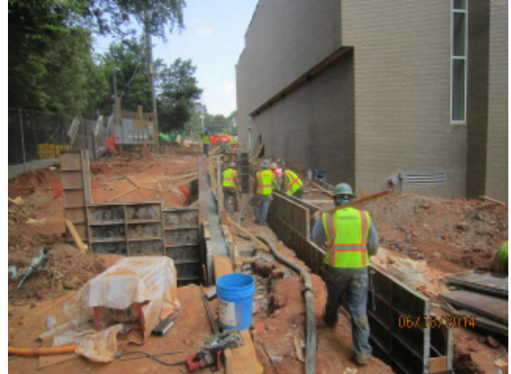
Pouring Site wall 'A' and Courtyard wall
