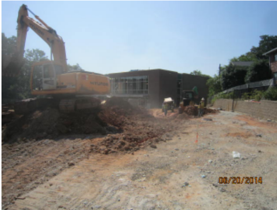
Grading at existing parking lot
