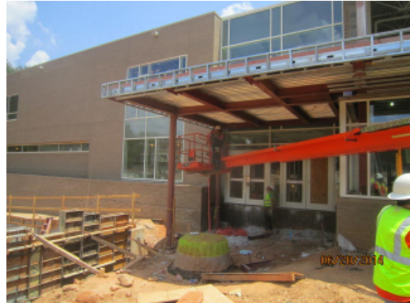
Aluminum Doors installed and gutter framed
