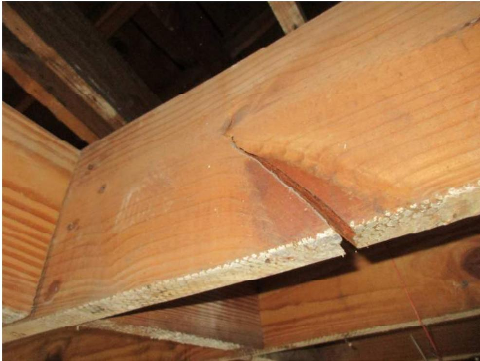
Photo 29: Typical Cracked Ceiling Joist
