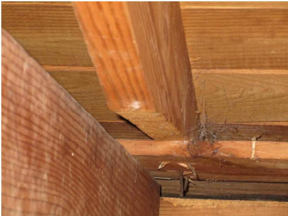
Photo 22: No Positive Connection at 1949 Roof Rafter-to-Exterior Wall Connection. Ceiling Joists and Roof Rafter Visibly Misaligned.
