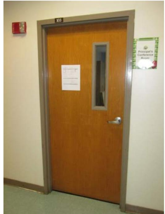
**Description:** Existing solid wood doors and door hardware throughout the facility appears to be functioning properly. The existing classroom locks are not up to date with the latest lockdown procedures.
