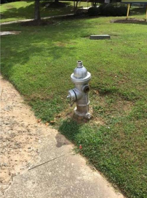
**Description:** According to Assessment report existing water line was installed in 1940 with 50 year service life. Was only able to locate one (1) hydrant on site which is in the front of school in r/w
