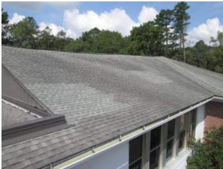
**Description:** The roof structure of Building #2030 is originally constructed in 1940 and is now failing in multiple locations.
