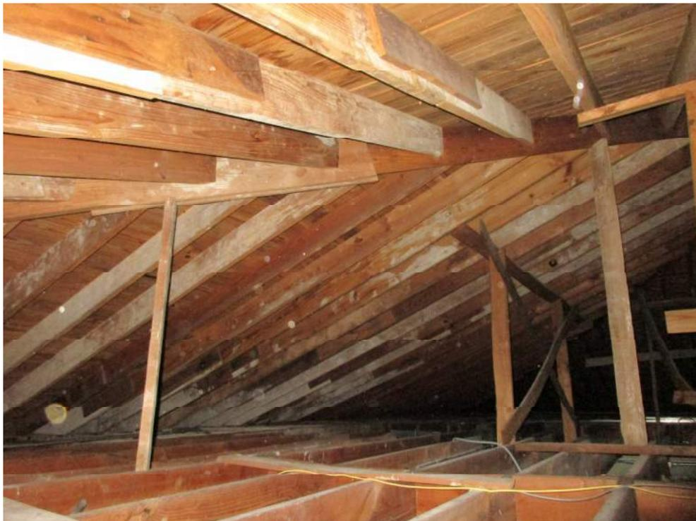
Photo 12: Typical 1949 Roof Structure Members with Visible Stains from Use as Concrete Formwork
