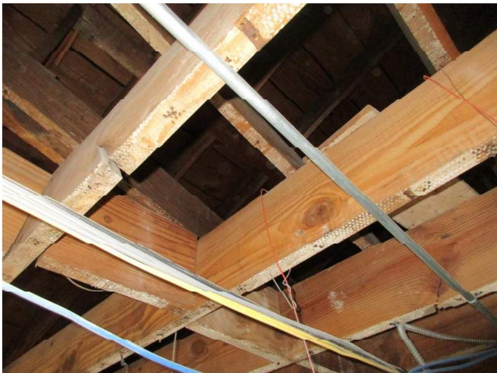
Photo 30: Typical Cracked Ceiling Joists
