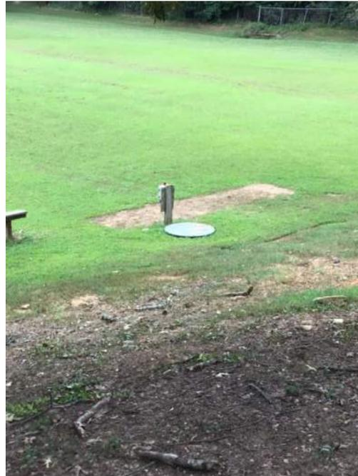
**Description:** According to Assessment report existing sewer system was installed in 1940 with 50 year service life. According to the achieved survey from 1991 the existing sewer line is 8" clay pipe. At time of visit we observed what appears to be a lift station down in field. This life station most likely pumps the building sewer flows around the existing building to the existing sewer system in the r/w
