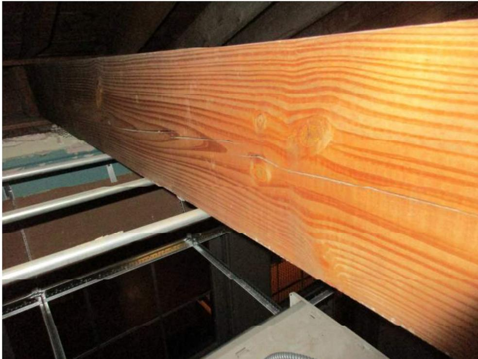
Photo 31: Typical Split Ceiling Joist
