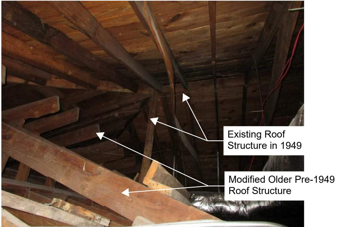
Photo 1: Existing Pre-1949 Roof Structure Additions
