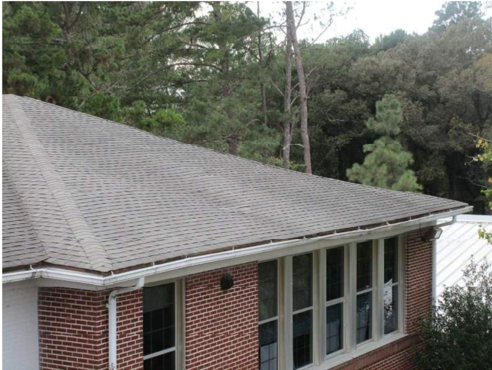
Photo 7: Visible "Sagging" of Northeast Classroom Roof
