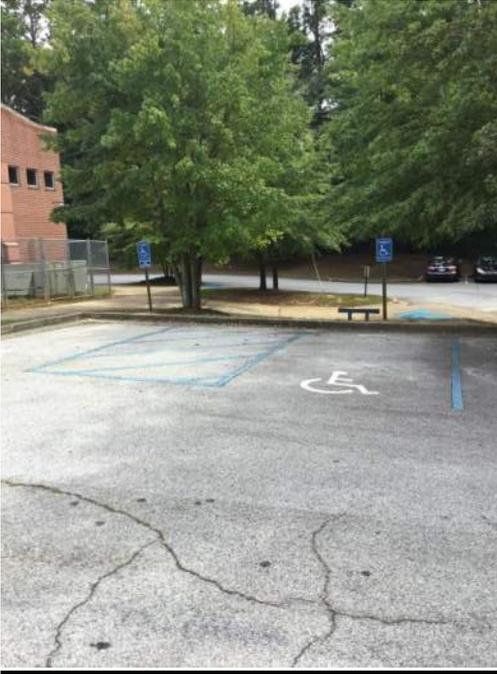
**Description:** ADA striping not complaint with code. The 3<sup>rd</sup> ADA space needs to have a striped landing and doesn't appear to be less than 2% slope in all directions
