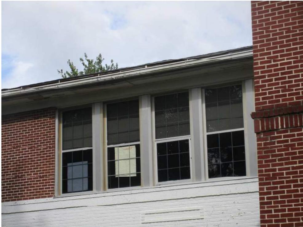
Photo 23: Bowed Window Header at Southwest Classroom Caused by Roof Lateral Thrust at Structurally Inadequate Roof-to-Wall Connections
