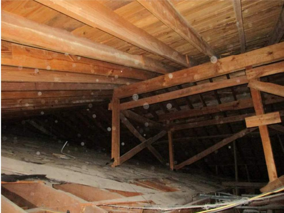
Photo 5: Existing 1949 Roof Structure Addition Built Atop Pre-1949 Structure (Looking South From Northeast Classroom)
