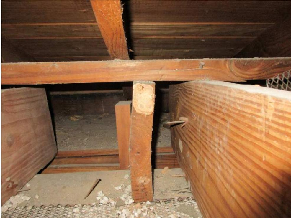
Photo 19: Cracked Pre-1949 Roof Rafter-to-Exterior Wall Connection. Ceiling Joists and Roof Rafter Visibly Misaligned.
