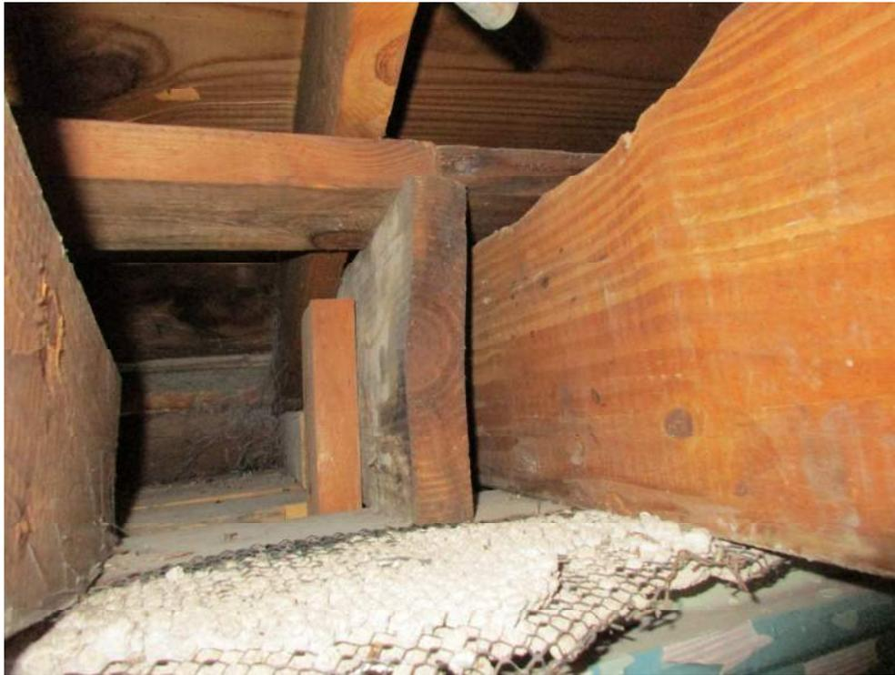
Photo 21: Water Damage and Member Bending at Pre-1949 Roof Rafter-to-Exterior Wall Connection. Ceiling Joists and Roof Rafter Visibly Misaligned.
