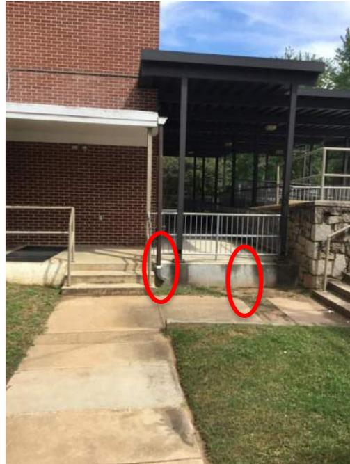
**Description:** Erosion in courtyard and damaged yard drain
