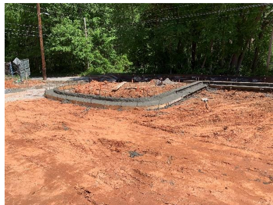
East Elevation Curb and Gutter
