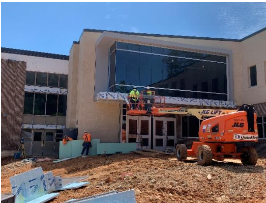
ACM Metal Panels
