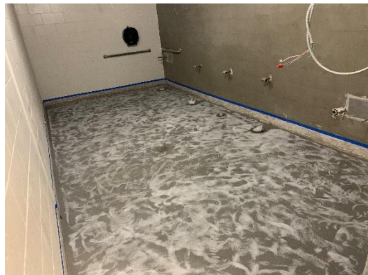
Epoxy Flooring in Gym Bathrooms
