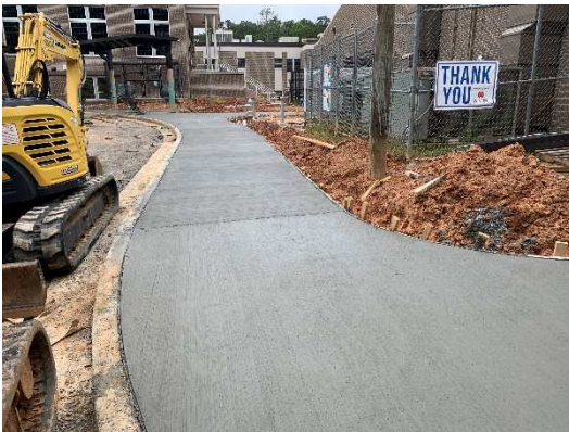
Sidewalks At The South Elevation
