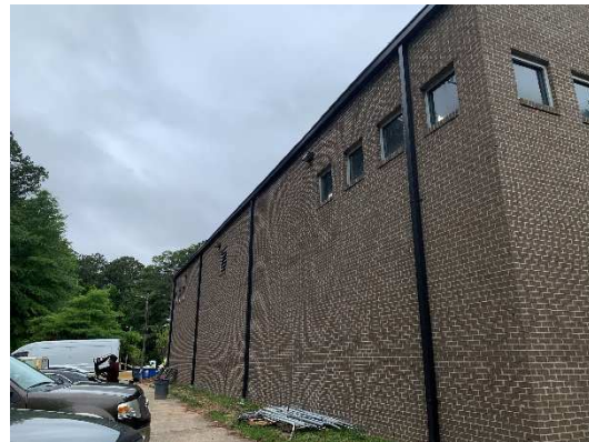
Roof Gutters And Downspouts At Building 2050
