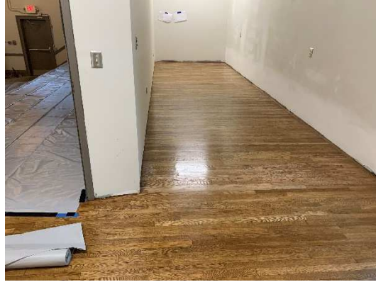
Media Center Wood Floor Staining
