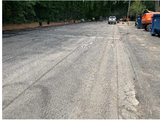
South Elevation Pavement Milling
