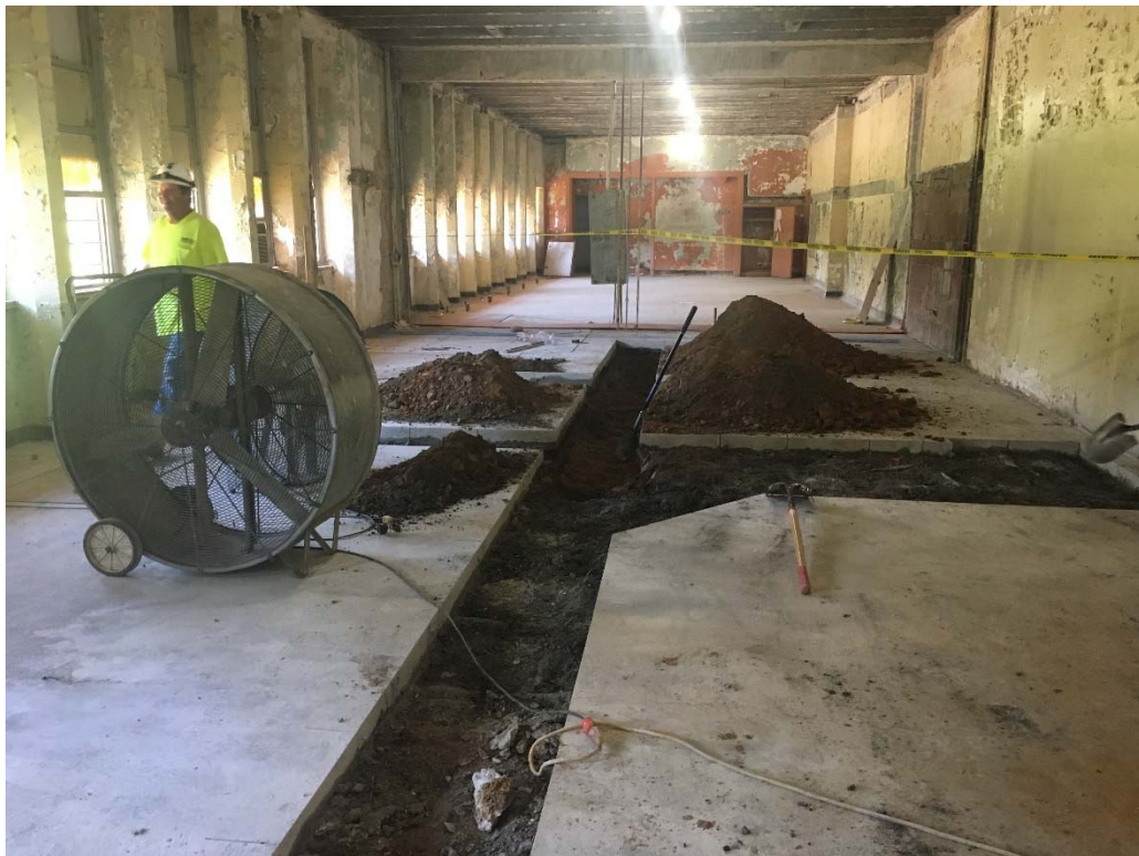
Plumbing trenches being cut on first floor
