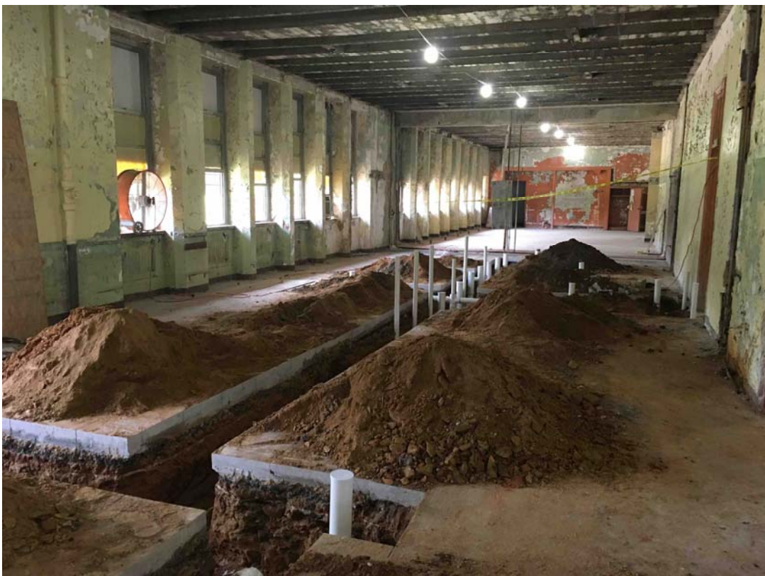
Plumbing piping being installed
