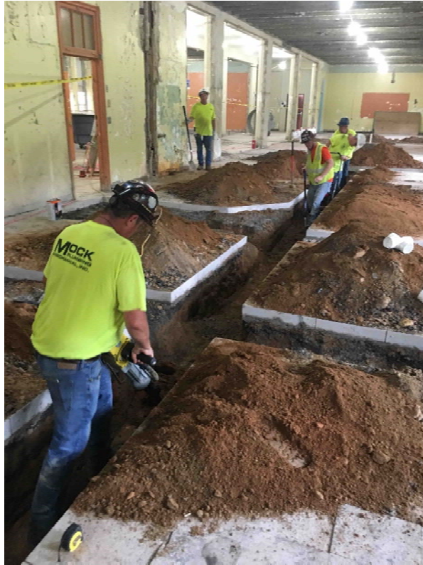
Plumbing piping being installed
