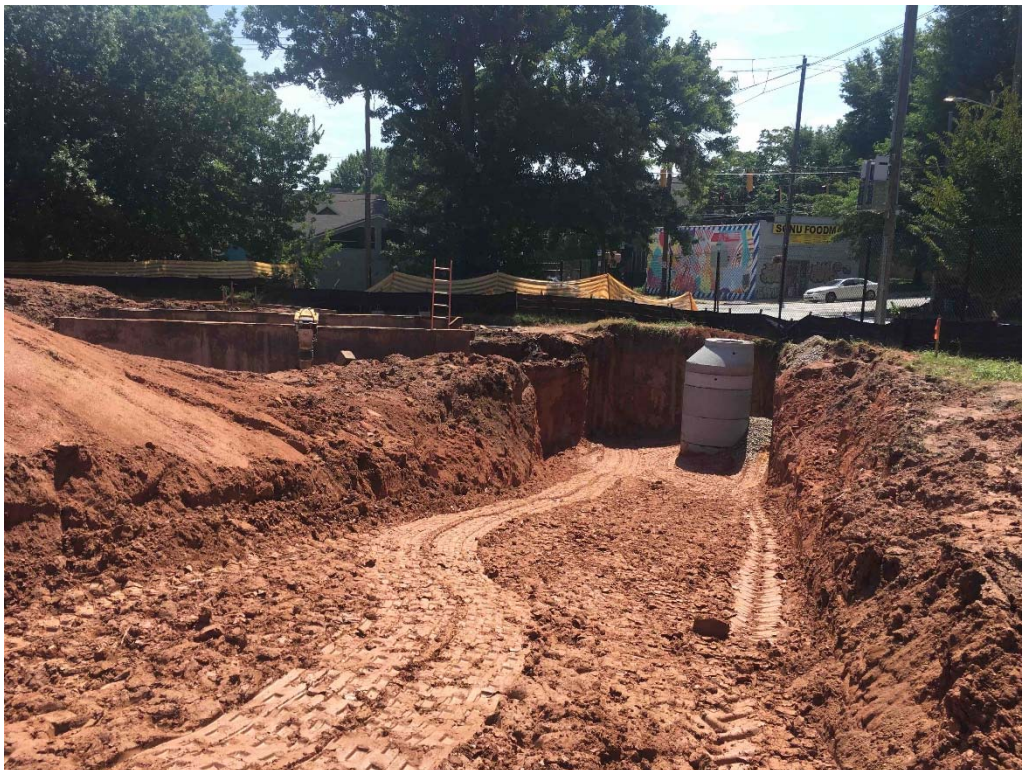
Storm structure at temp pond installed
