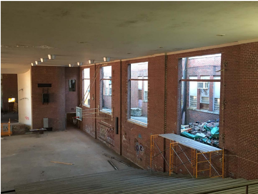
Gym windows being removed for restoration
