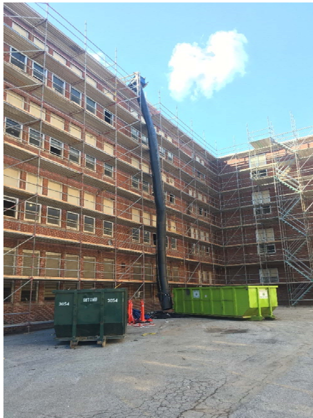
Roofing demo trash chute being installed on West Wing
