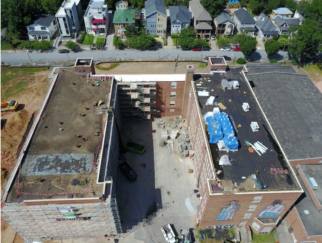
Roofing tear off on West Wing
