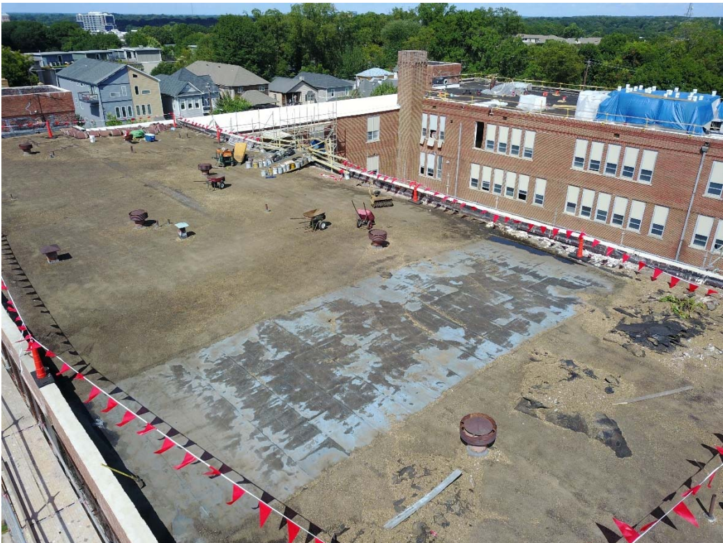
Roofing tear off on West Wing
