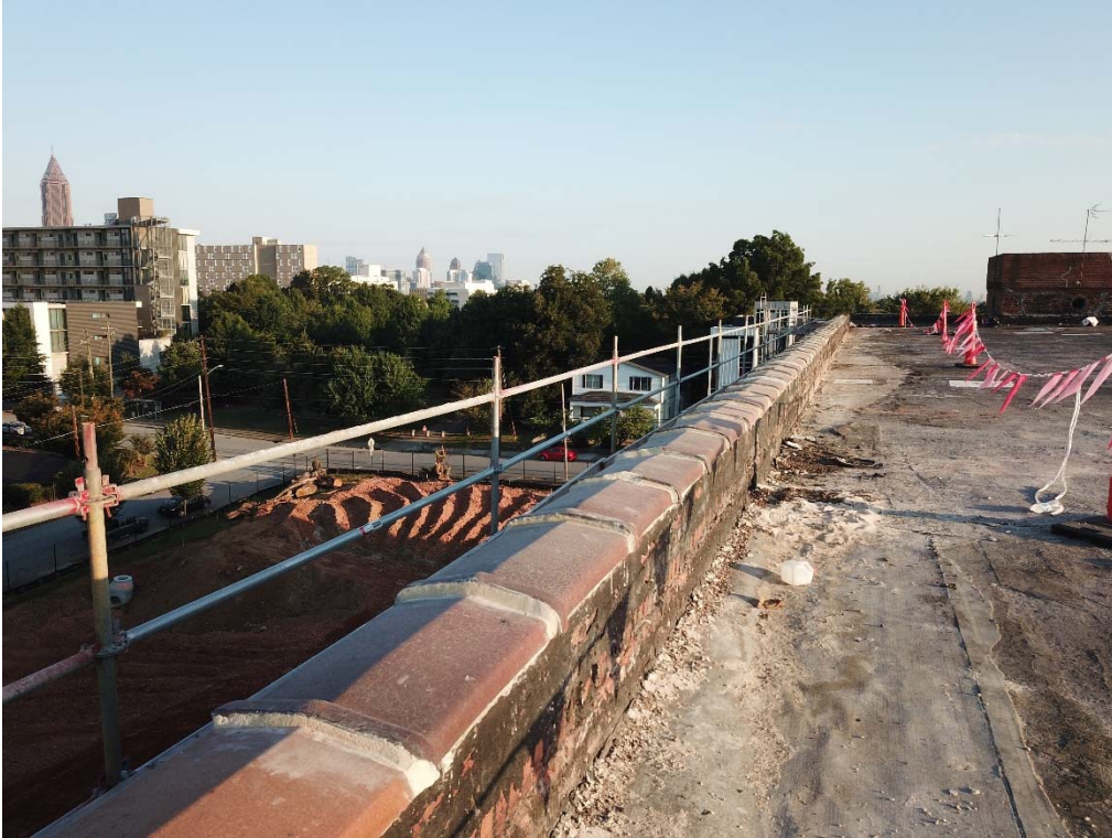
Coping being installed on West Wing
