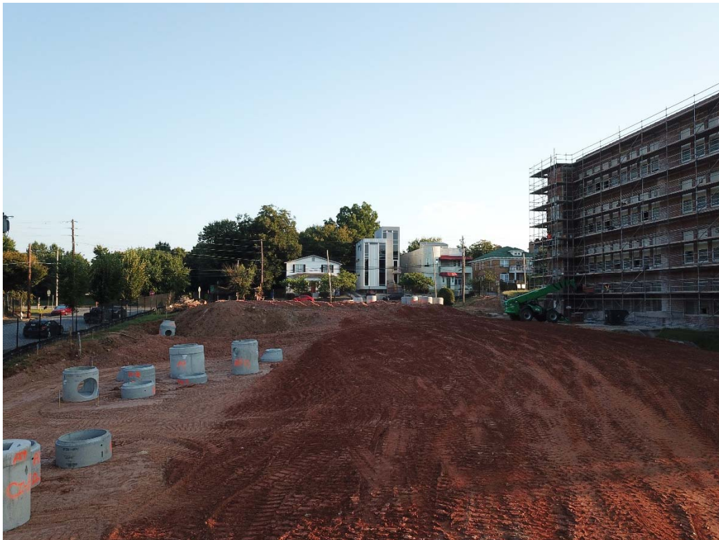
Preparing subgrade for addition on West side of property
