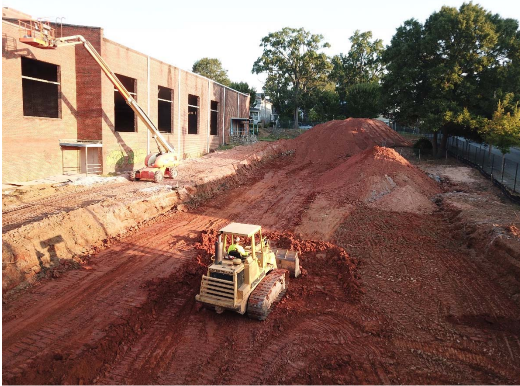
Preparing subgrade for addition on West side of property
