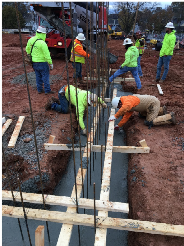
Concrete footers being poured
