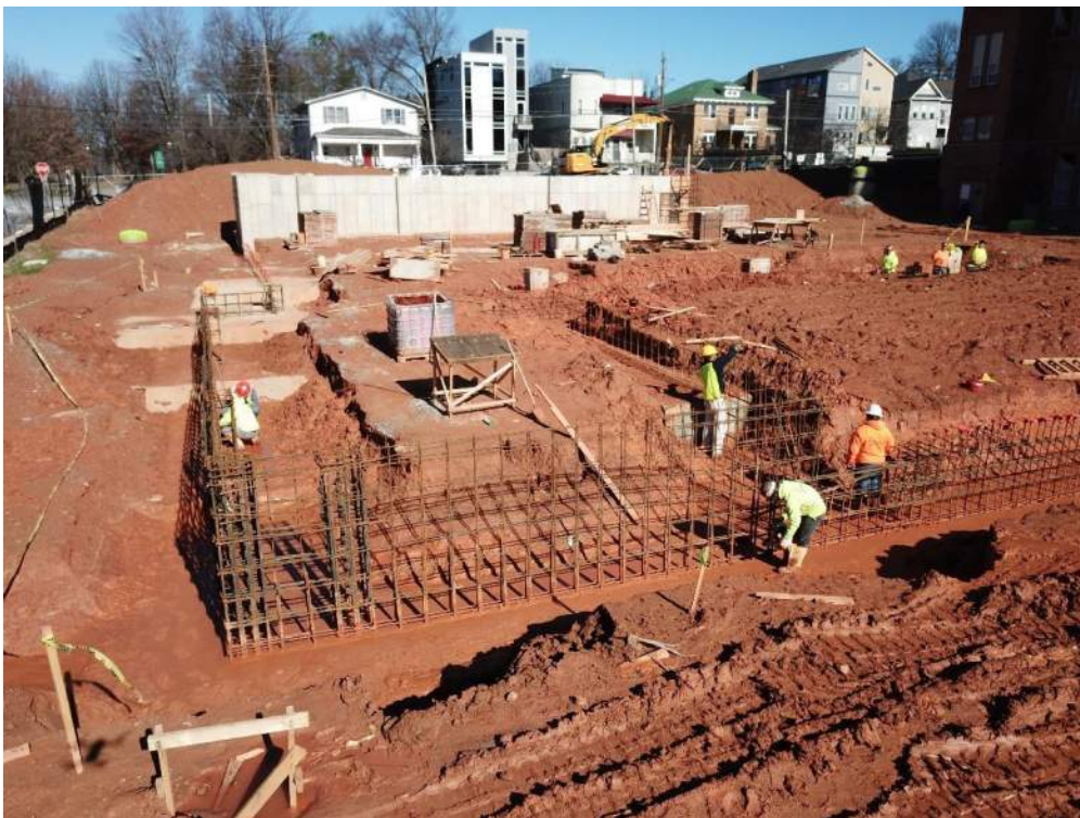
Rebar installed for foundation wall South side of new addition
