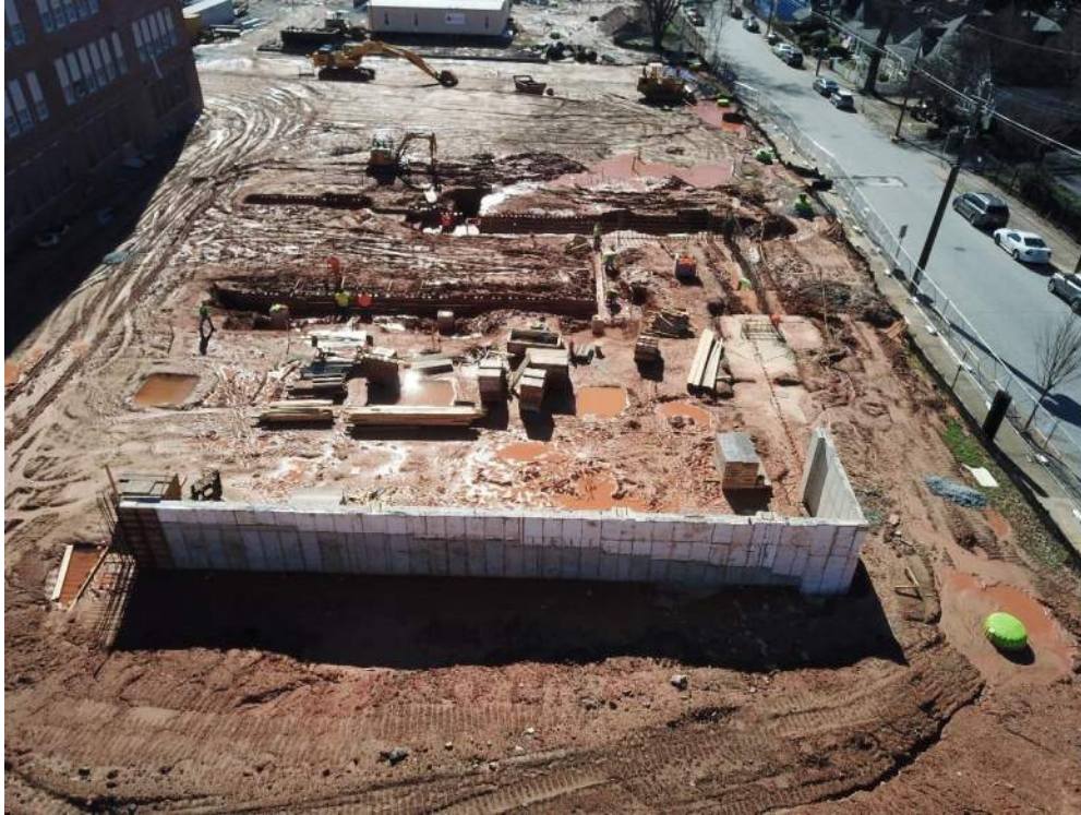
Aerial view of Area 1 concrete footers and retaining wall facing North
