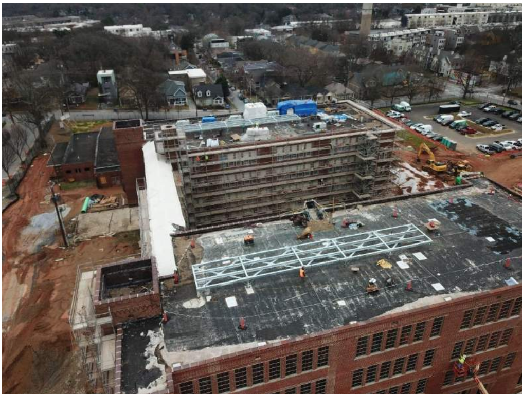
Roof top unit steel being installed
