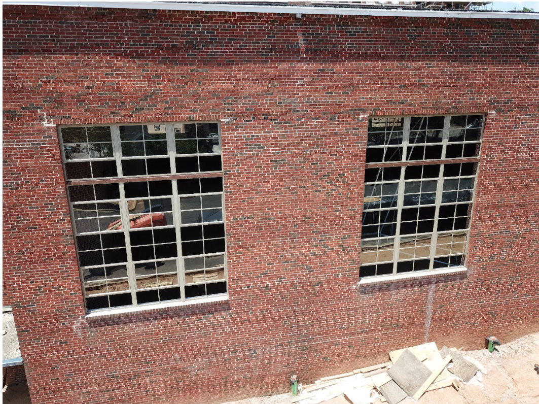
Existing Building Gym Restoration Window Installation
