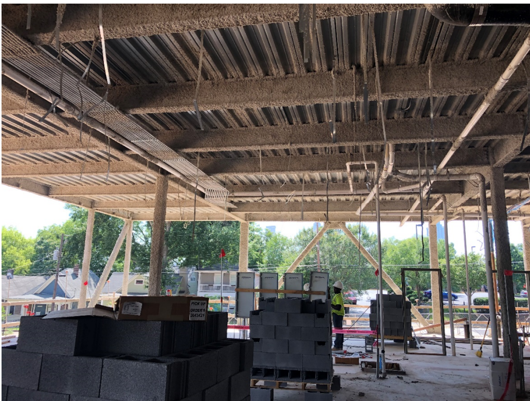
Spray fireproofing being installed in Area 5
