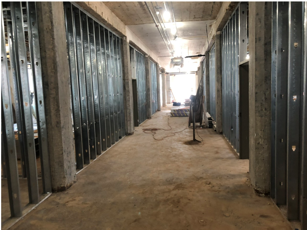
Interior Metal Stud Installation Continuing
