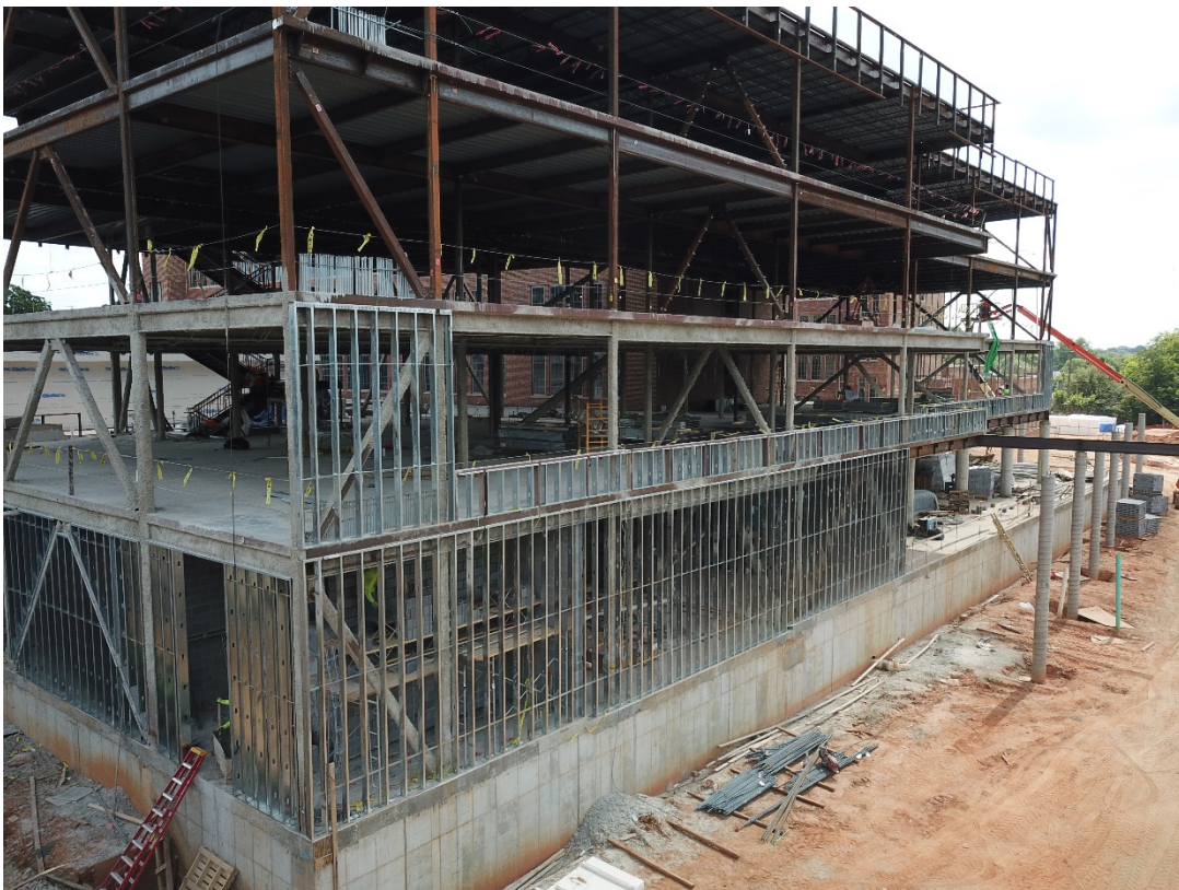
Area 5 Exterior Metal Stud Installation
