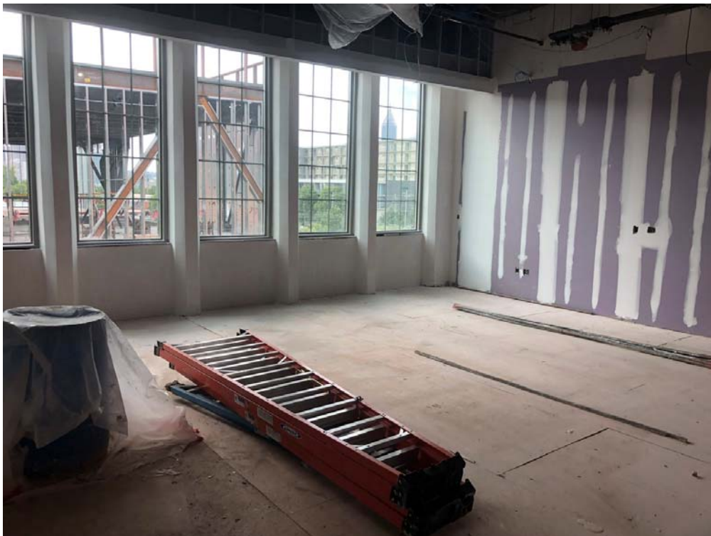
West Wing Gyp and flooring Progress
