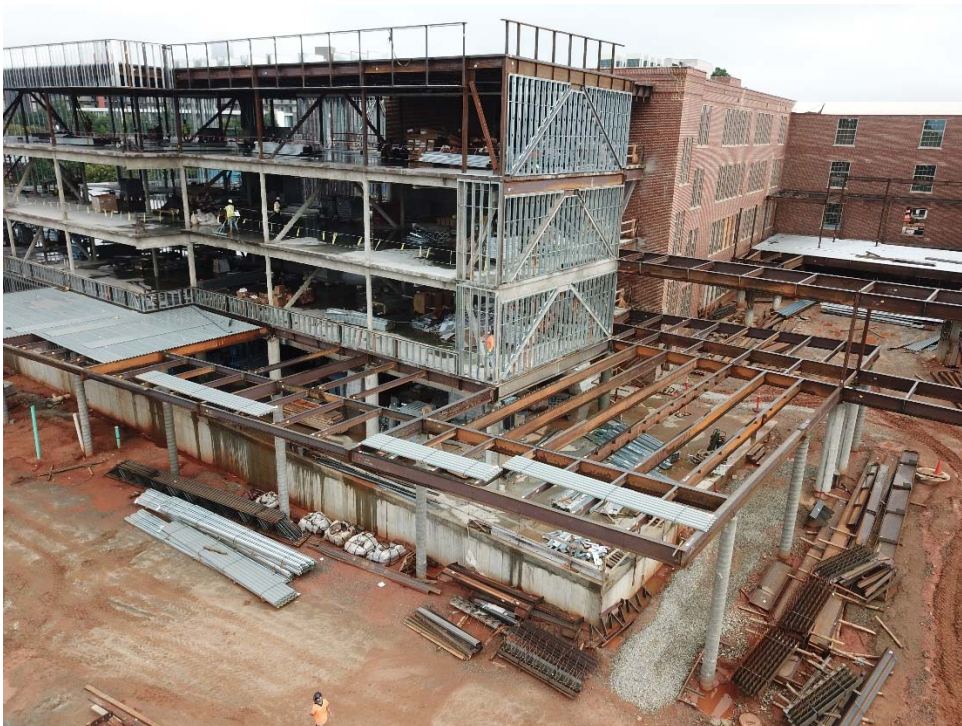
Area 5 Metal Stud and Canopy Installation
