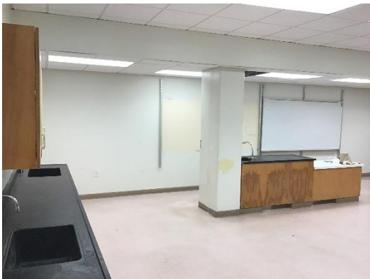
Existing Second Level Classroom
