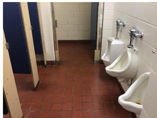
Existing Second Floor Bathroom Fixtures
