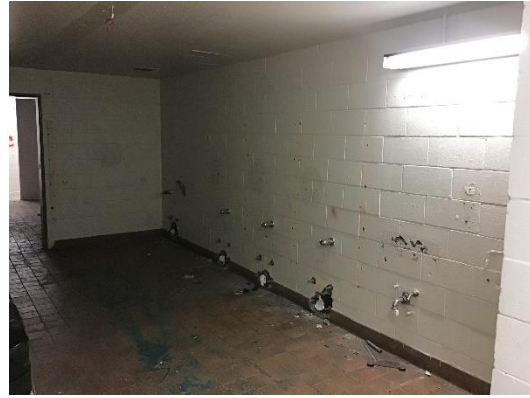
Gymnasium Bathroom Partition Demolition
