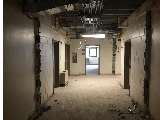
Second Floor Hallway CMU Wall Demolition
