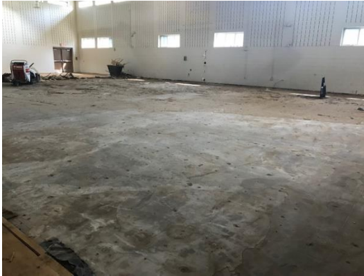
Gymnasium Flooring Demolition
