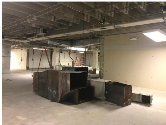
Second Floor Mechanical Duct Demolition
