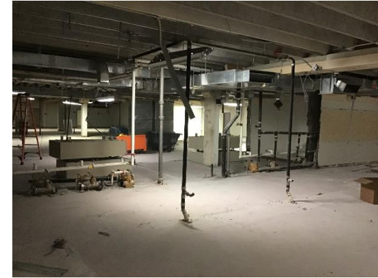
Second Floor Plumbing Piping Demolition
