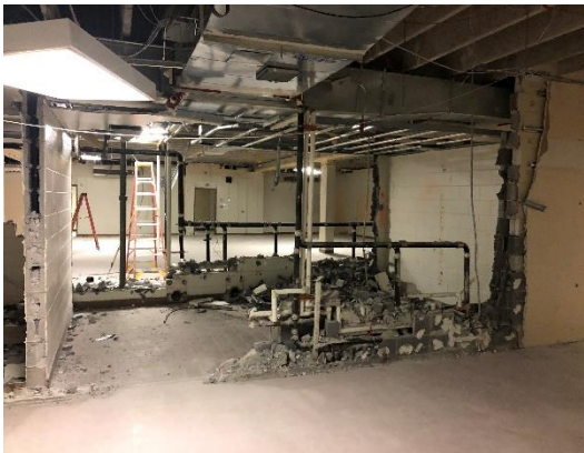
Second Floor CMU Wall Demolition
