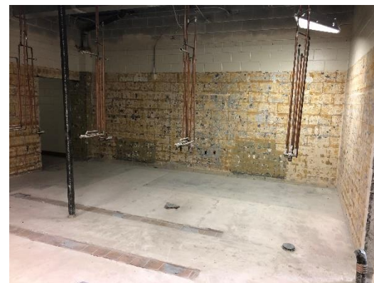
Gymnasium Showers Partition Demolition
