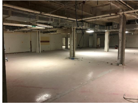
First Floor Hallway Partition Demolition
