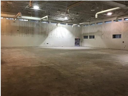
Gymnasium Flooring Demolition
