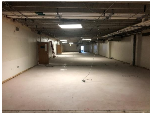
First Floor Classroom Partition Demolition
