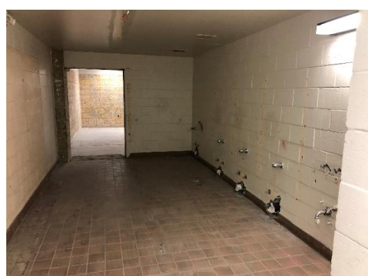
Gymnasium Bathroom Partition Demolition
