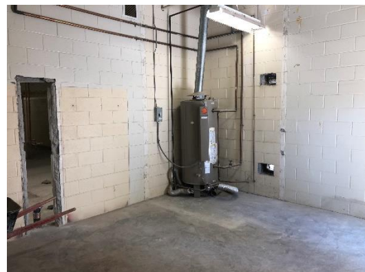
Gymnasium Boiler Room Partition Demolition
