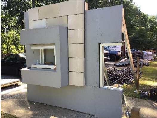
Front View of Exterior Mockup
