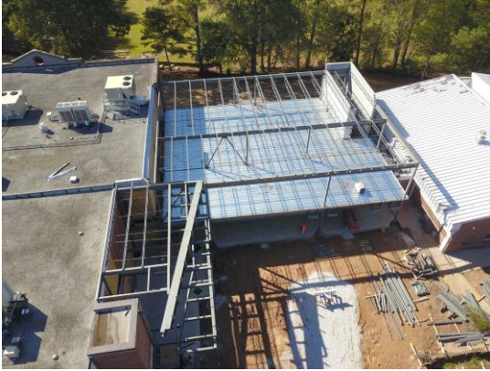
Building Addition Aerial View
