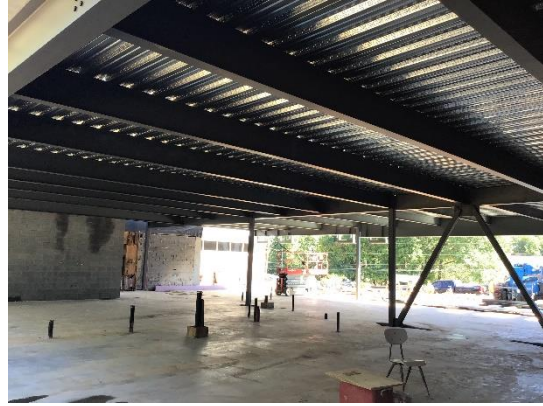
Building Addition Floor 2 Decking
