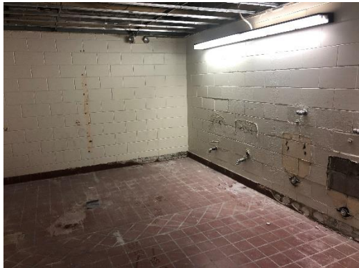
First Floor Bathroom Partition Demolition
