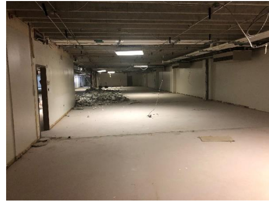
First Floor Classroom Partition Demolition
