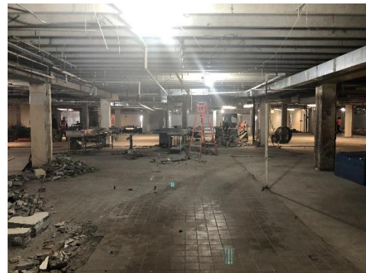
Cafeteria Kitchen CMU Wall Demolition
