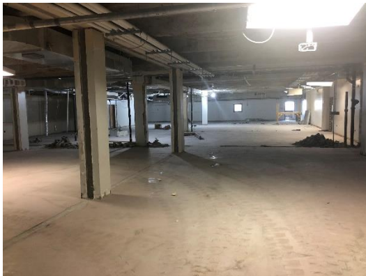
First Floor Hallway Partition Demolition
