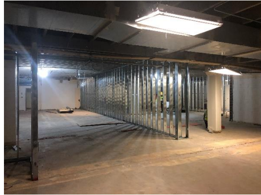
Second Floor Classroom Framing
