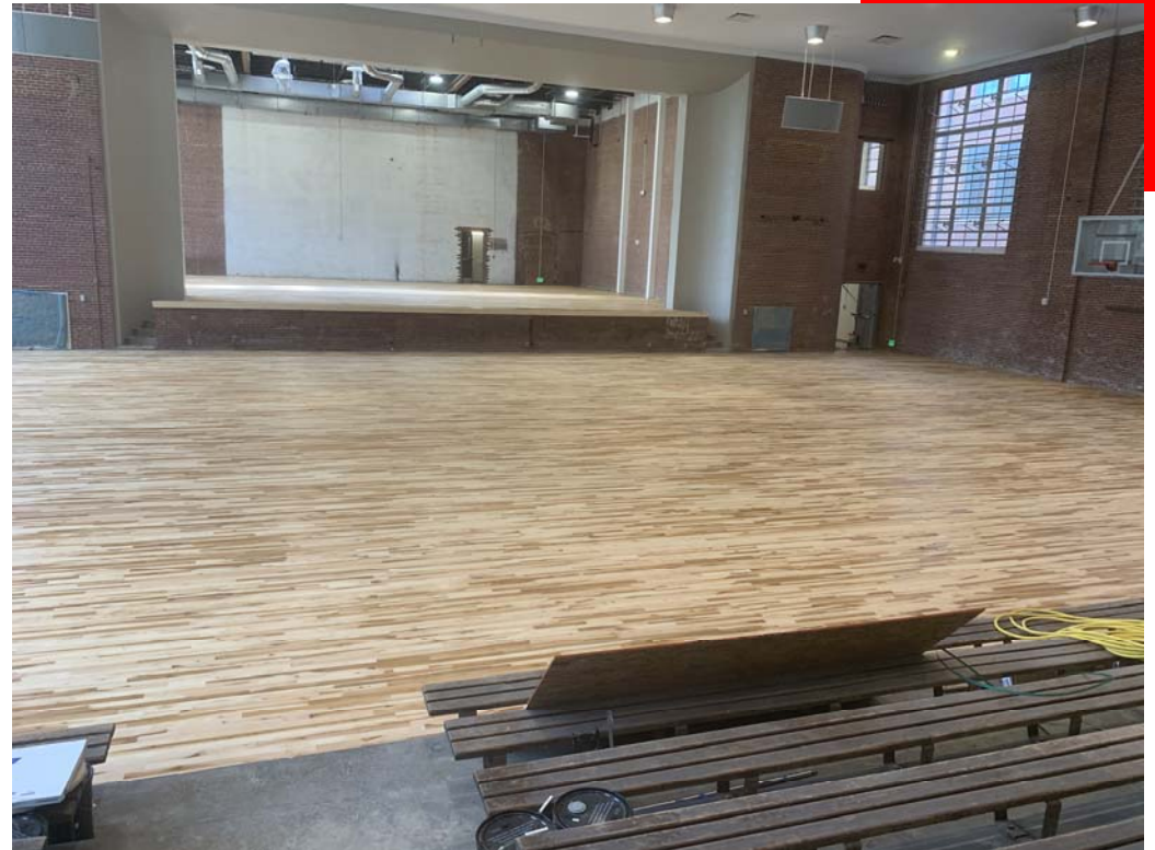
Existing gym wood floor install
