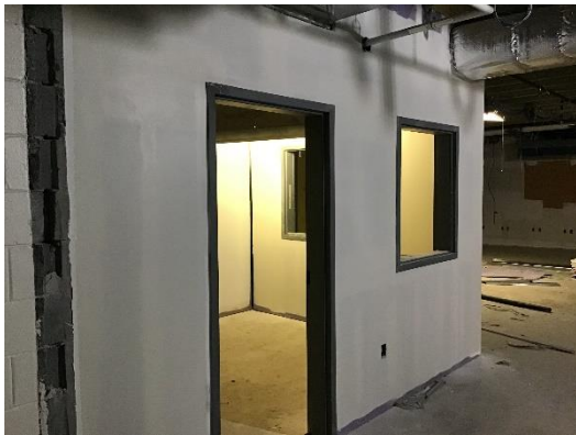
Drywall Prep for Paint at Graphics Lab
