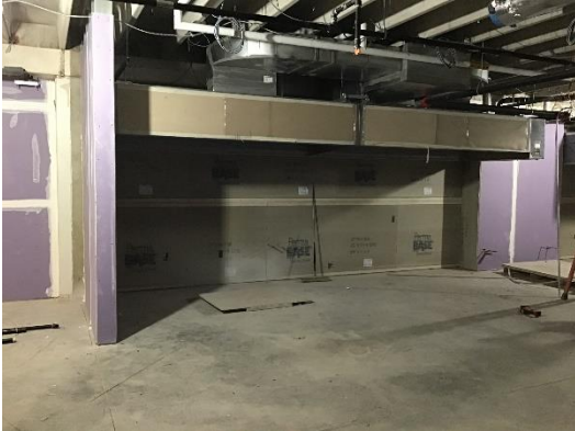
Kitchen Hood Installation at Culinary Arts Lab
