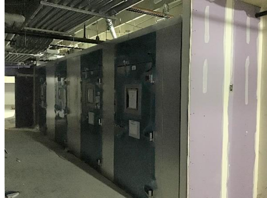
Walk-In Cooler/Freezer Installation
