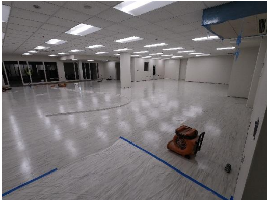
VCT Flooring Installed at Graphics Lab 252
