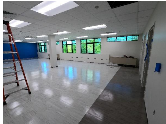
VCT Flooring Installed at Level 02 Classroom
