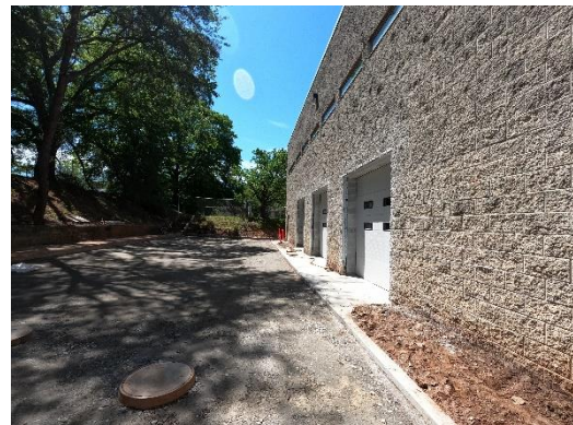
Curbs and Flatwork Installed at Auto/Aviation Labs
