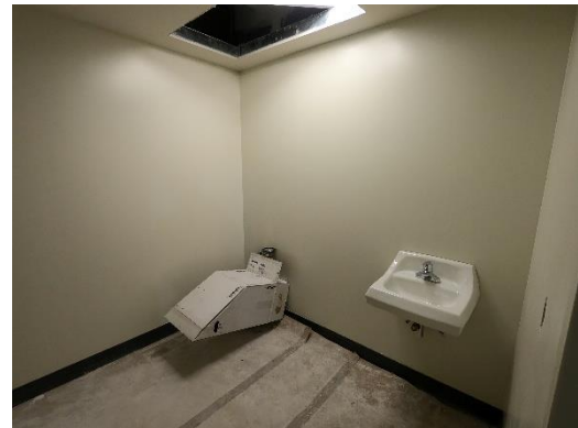
Level 01 Restroom Plumbing Fixtures Installed
