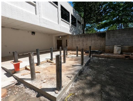
New Dumpster Pad Installed
