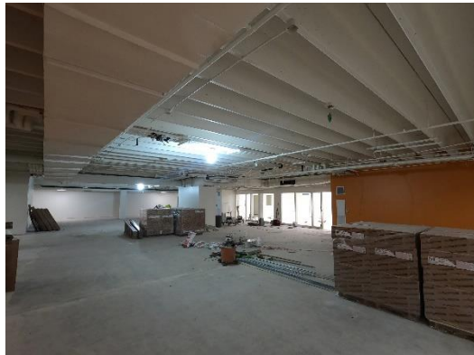
Exposed Ceiling Painted at Commons 201
