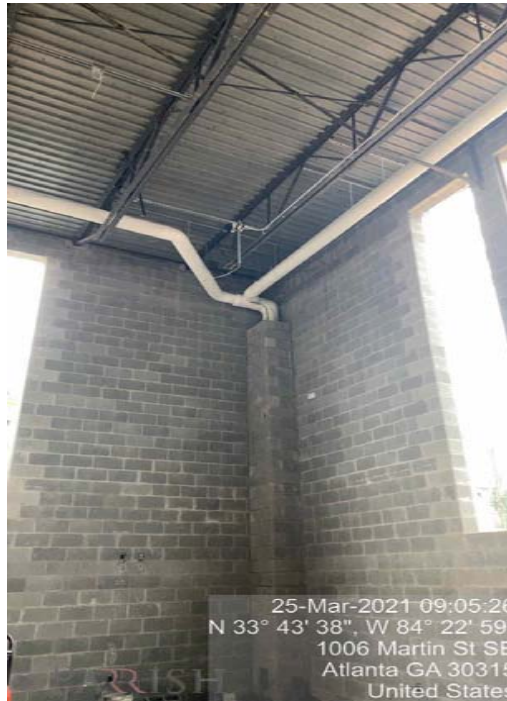
Roof drain installation
