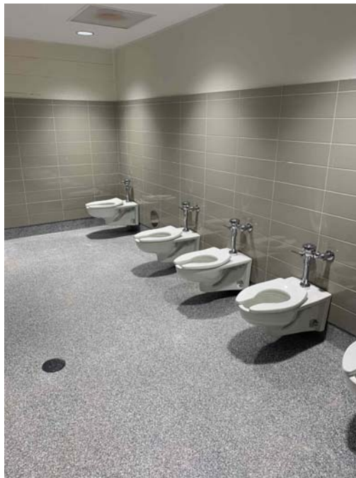
Plumbing fixture and wall tile installation
