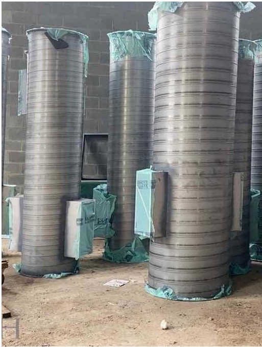
Spiral duct delivery
