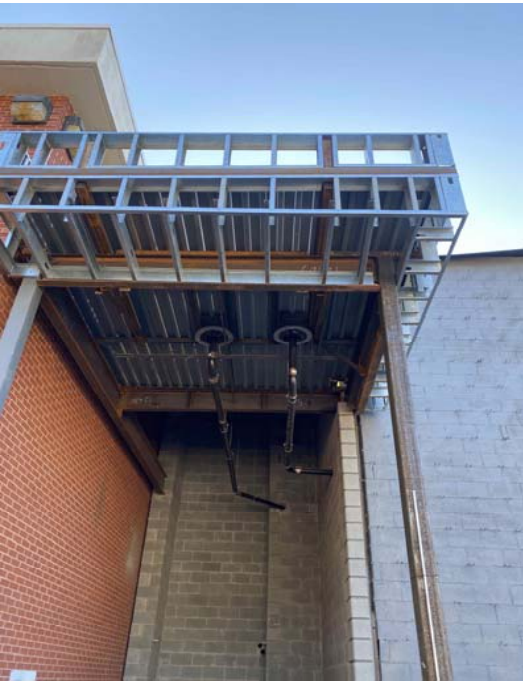
Parapet framing
