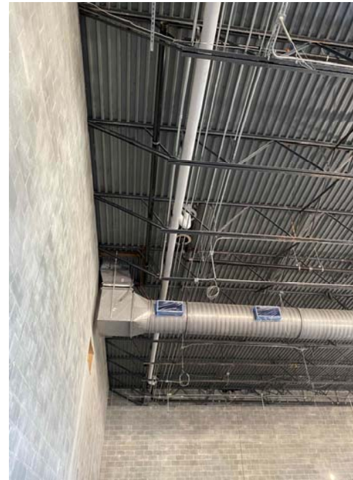
New gym ductwork
