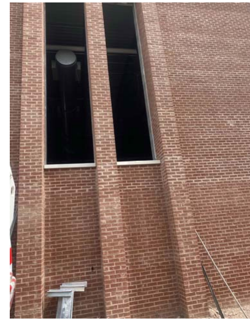
Precast concrete installation
