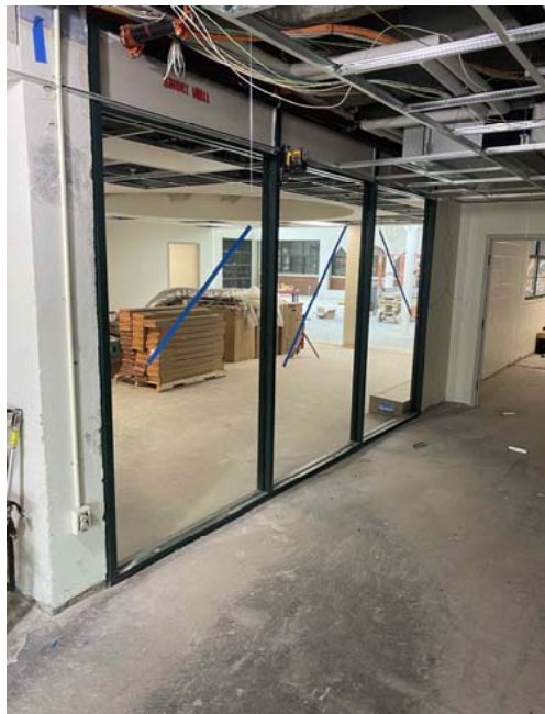
Glazing installation
