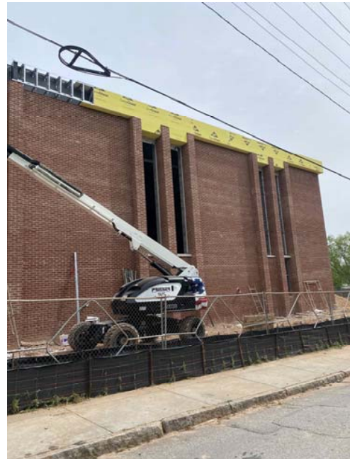
Gym soffit sheathing
