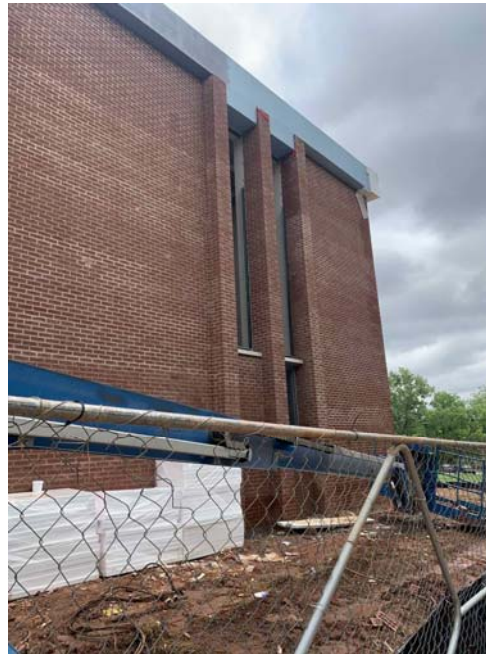
New gym EIFs installation
