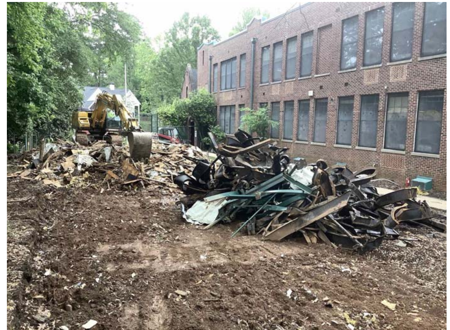
Portable trailer demolition
