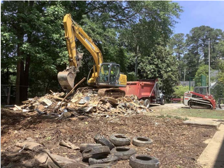
Portable trailer demolition
