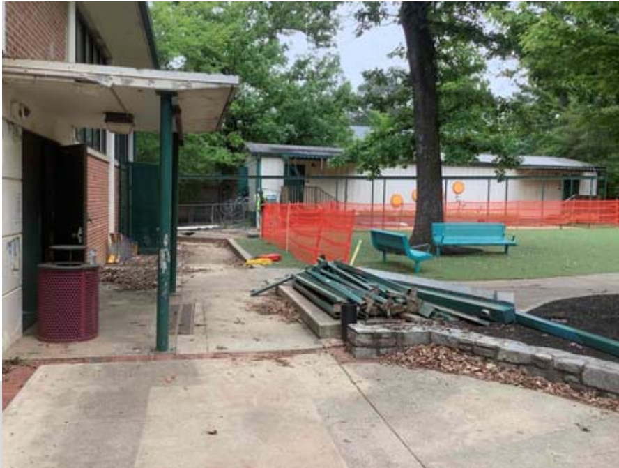
Aluminum walkway cover demolition
