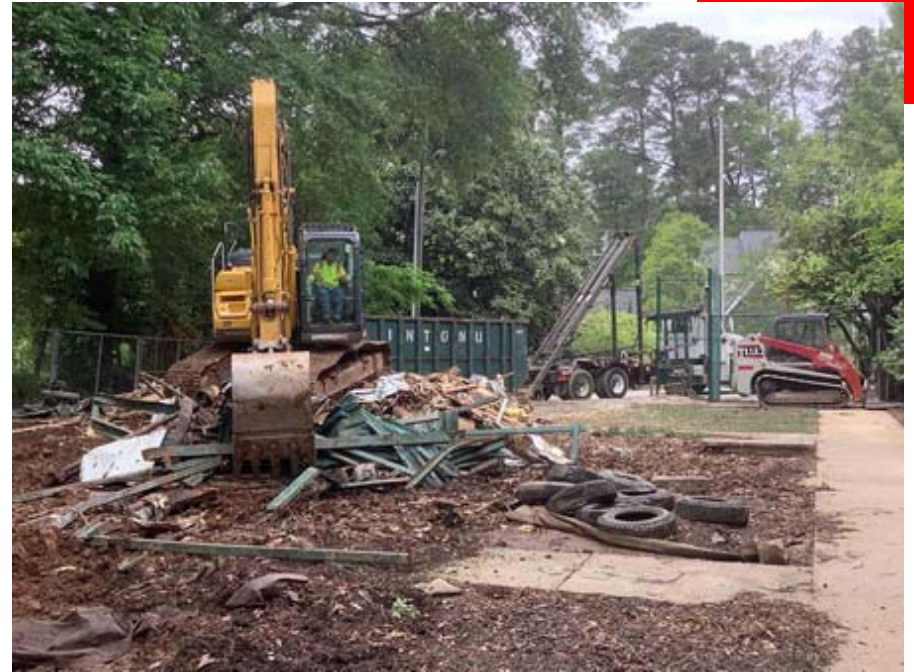
Portable trailer demolition
