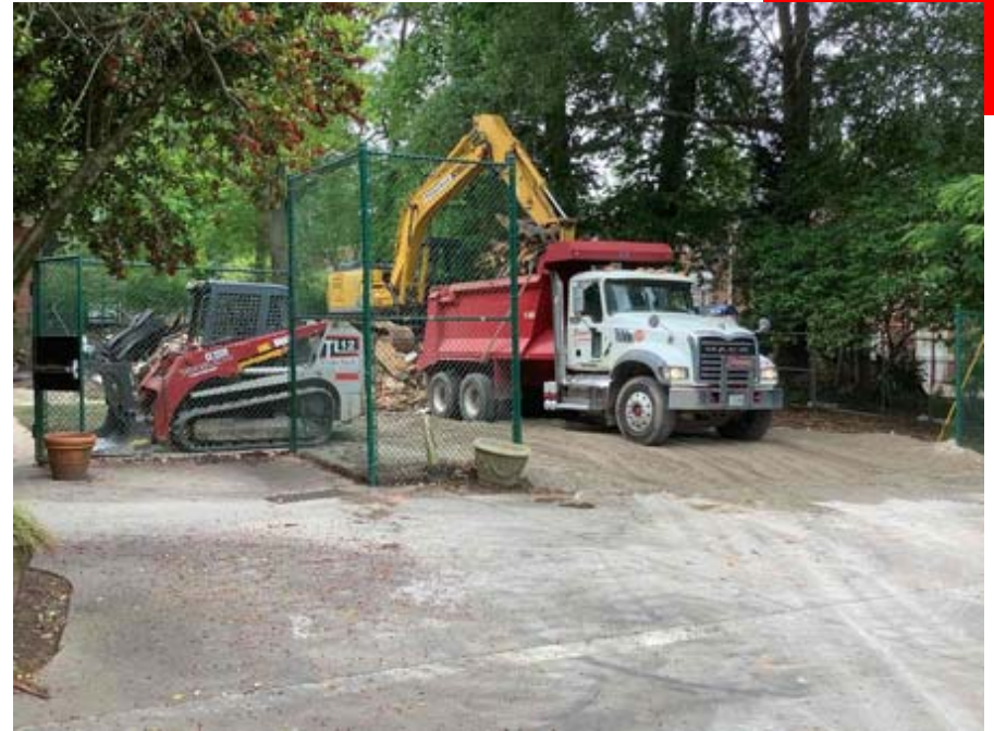
Portable trailer demolition
