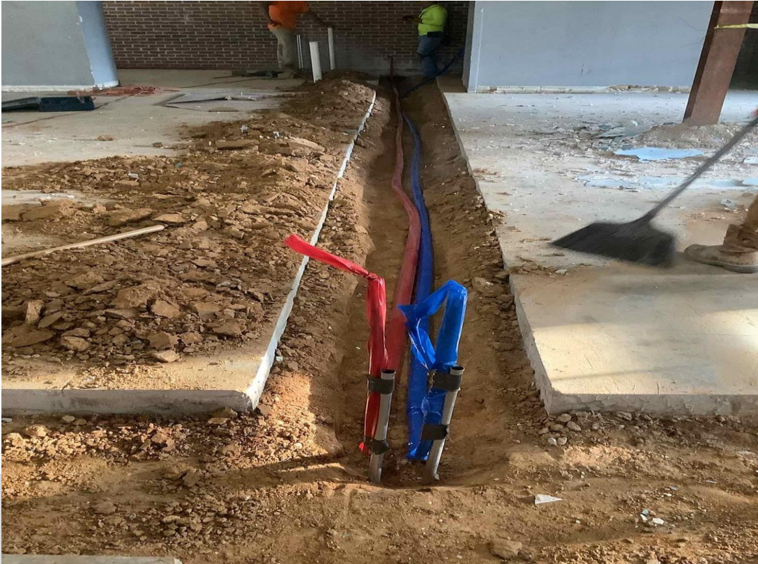
Hot and cold water piping
