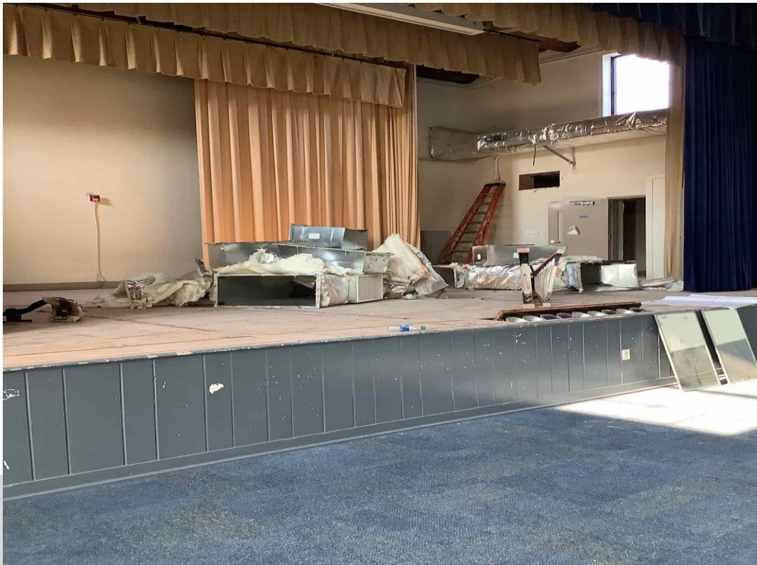
Mechanical demolition
