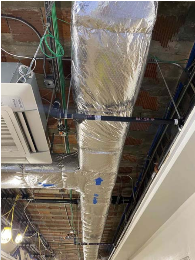
Fire sprinkler and HVAC rough-in
