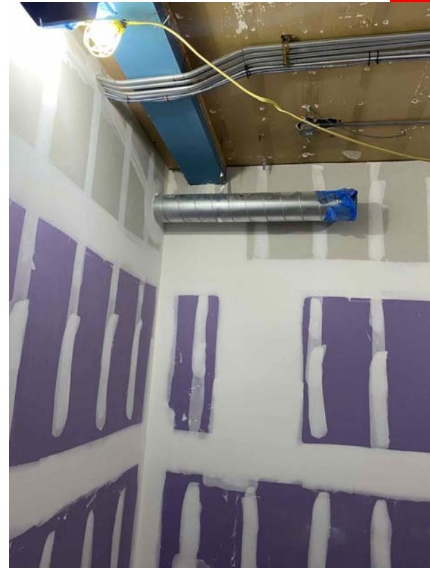
Drywall finishing and mechanical/electrical rough-in
