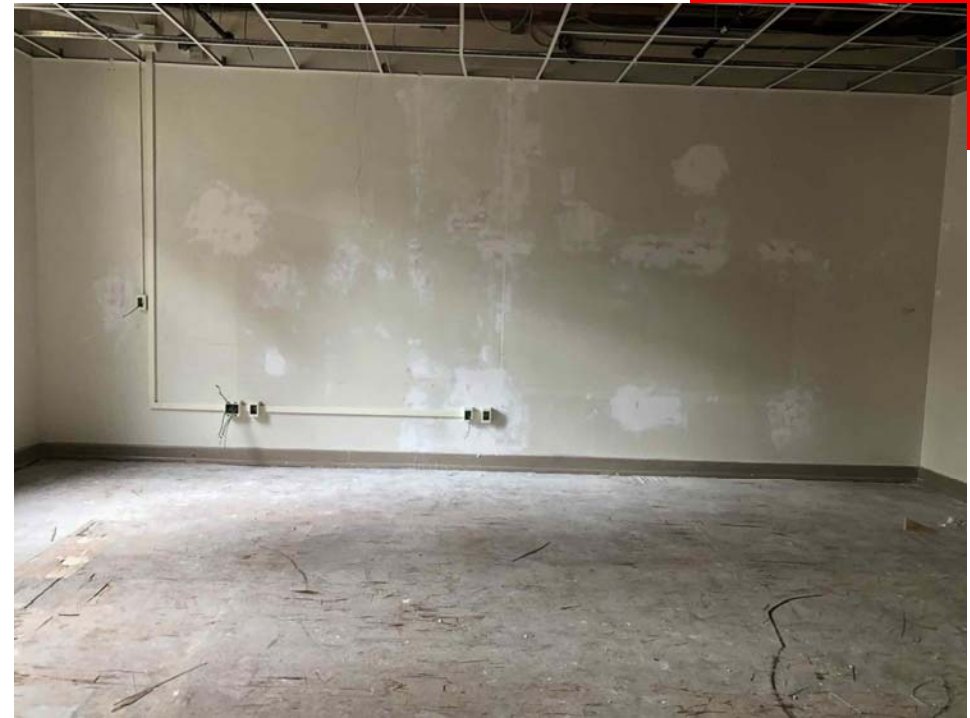
Plaster repair and wire mold installation
