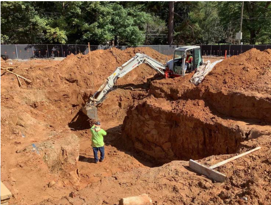
Excavation for new gym footings
