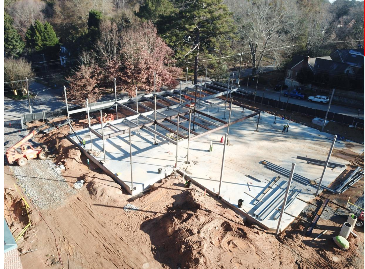
Structural steel installation
