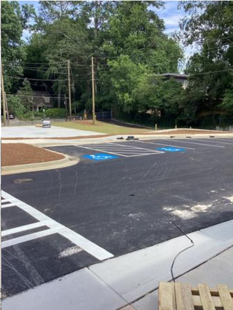
Asphalt striping installation
