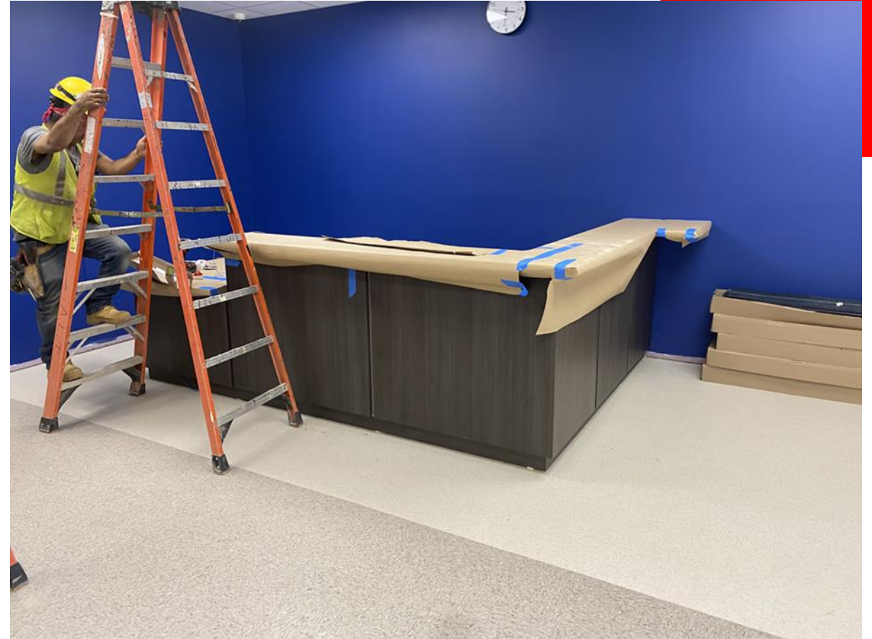
Reception desk installation
