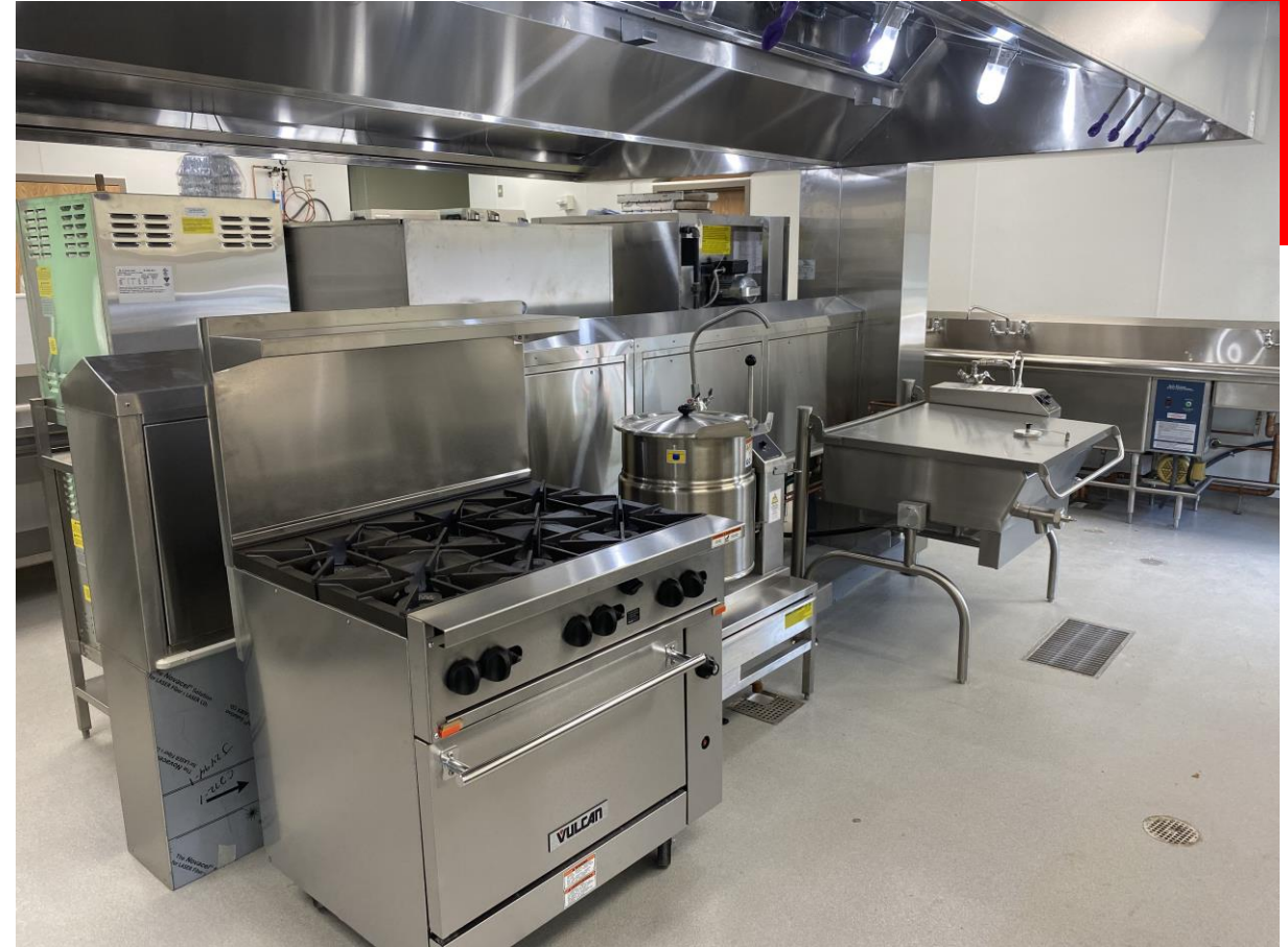
Kitchen equipment installation
