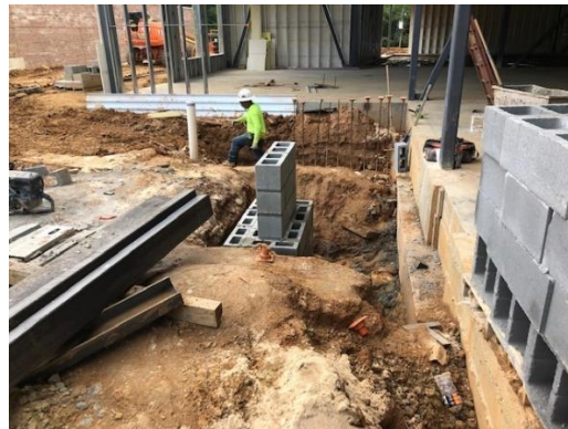
Masonry knee wall at YMCA
