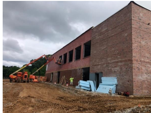
Metal Panel prep West Elevation at WPA
