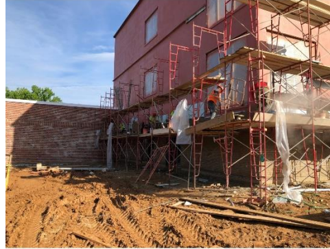
Brick at South Elevation at WPA
