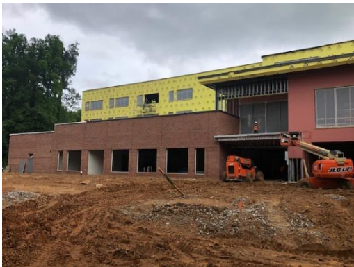
Sheathing and Air Barrier West Elevation at WPA
