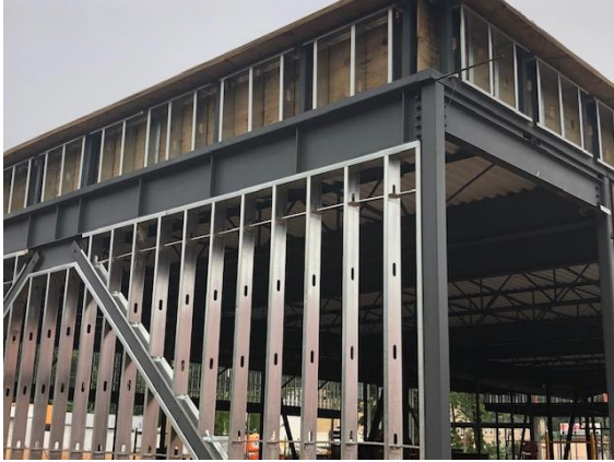
Parapet framing at the YMCA
