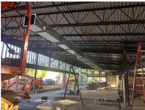
Ductwork install started at YMCA
