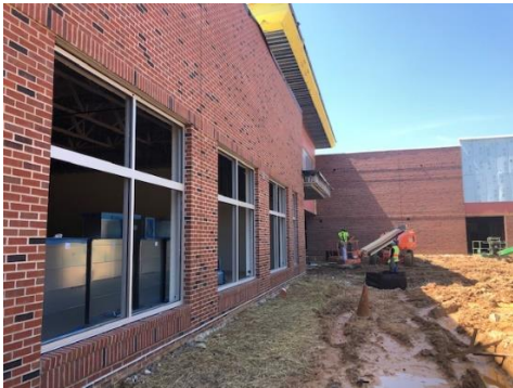
Cafeteria window frames install
