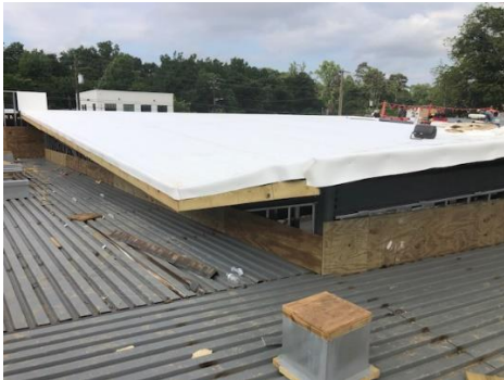
Roofing at the YMCA
