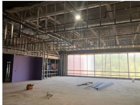
Media Center soffit framing
