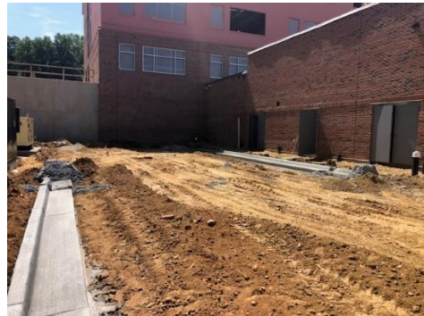
Curb and Gutter started on Bus Loop
