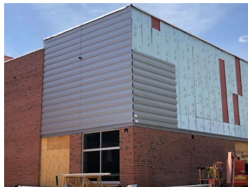
Metal Panel install at WPA
