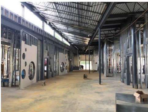
Interior framing at YMCA
