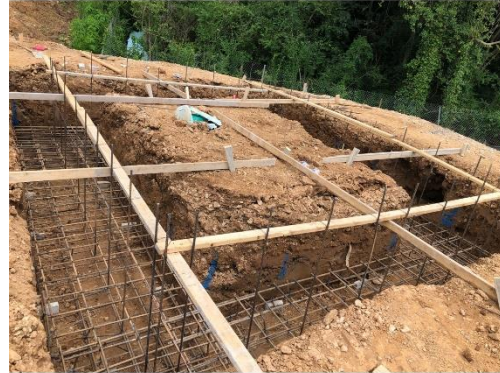
Dumpster pad footings at YMCA
