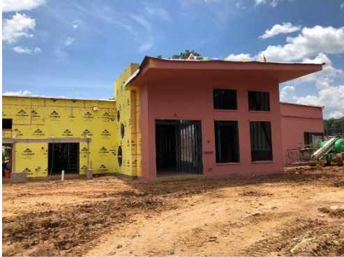
Vapor Barrier at YMCA
