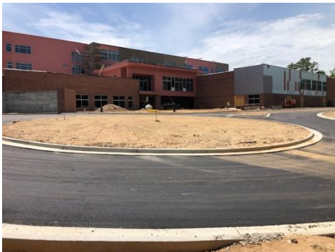
Binder complete at Bus Loop
