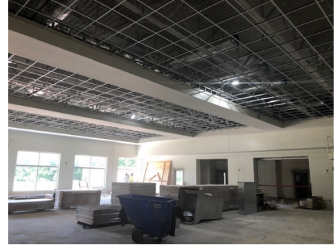
Drop in ceilings at Cafeteria area
