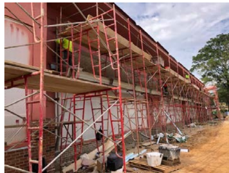
South Elevation at the YMCA
