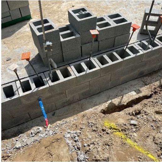
12" Foundation CMU Install
