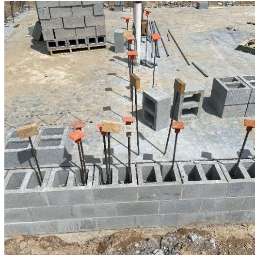
12" Foundation CMU Install
