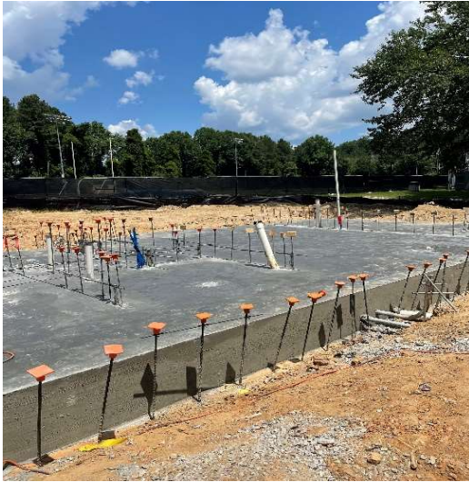
Slab On Grade South Elevation
