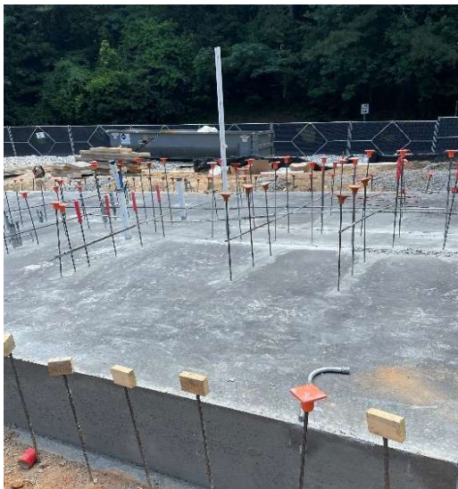
Slab On Grade West Elevation
