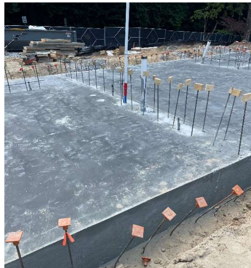
Slab On Grade North Elevation
