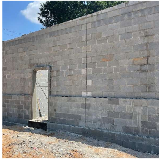
CMU East Elevation
