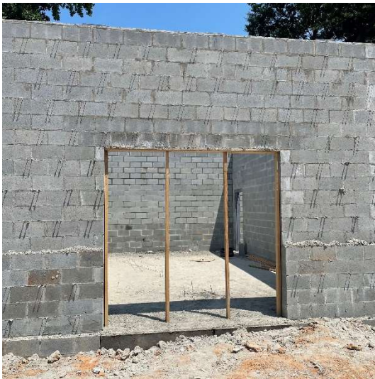
CMU At Overhead Door
