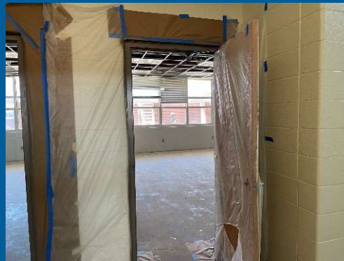
Door Frames 1 st coat of Finish Paint
