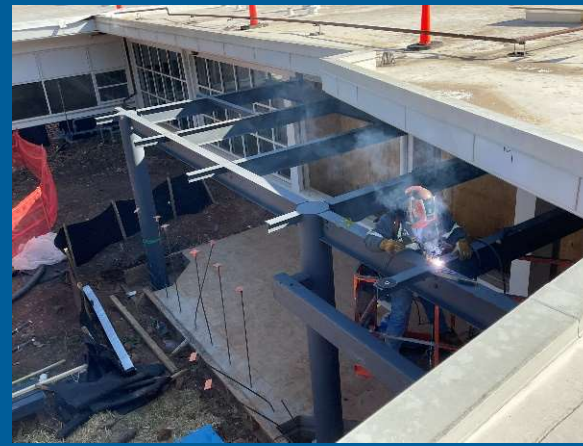
Vestibule Structural Steel Installed
