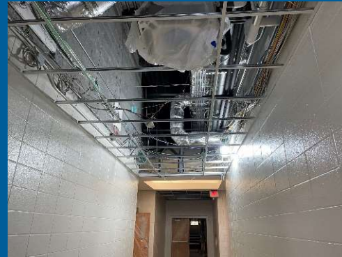
Ceiling Grid Installed in Areas B,C Hallways
