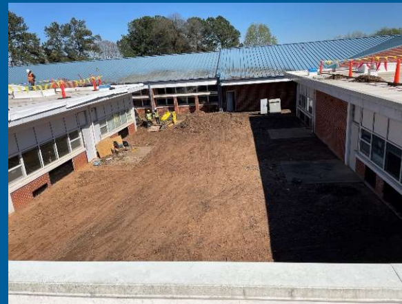
Grading and Clearing at Courtyard
