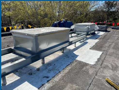
HVAC Rooftop Curbs Set at Cafeteria
