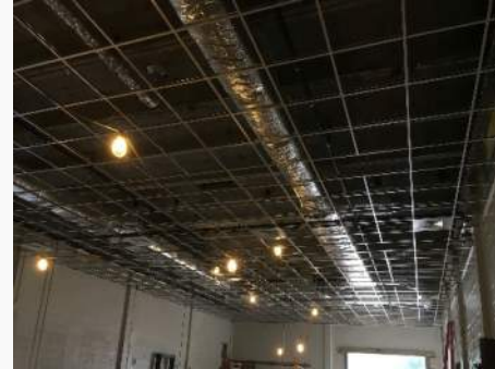
Ceiling Grid at Auditorium
