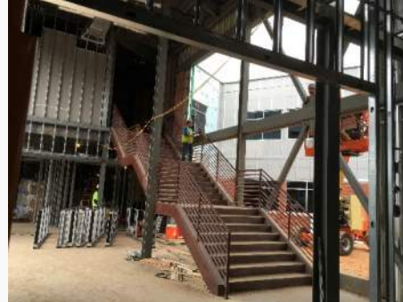
Installing Window Walls at Lobby
