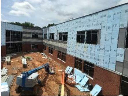
Windows & Metal Panels at Courtyard
