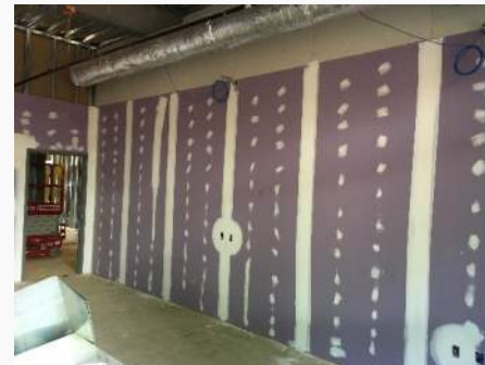
Drywall, Hang, Tape, & Finish
