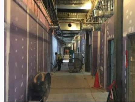
Drywall, Hang, Tape, & Finish
