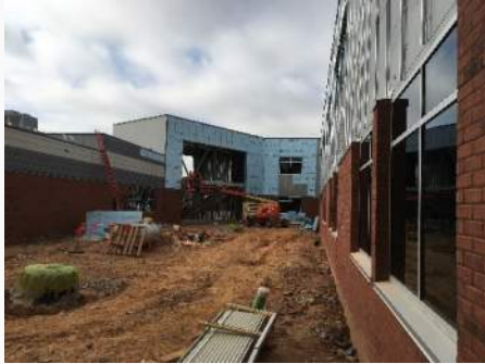
Windows & Metal Panels at Courtyard
