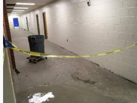
VCT Floor Leveling & Patch at Renovation
