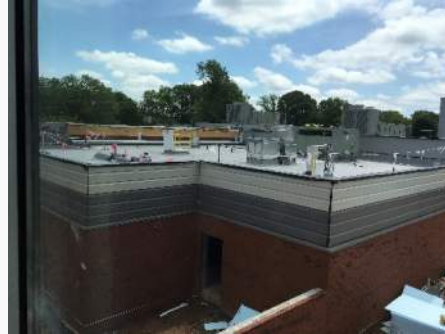
Metal Panels & Roof Top Equip. at Kitchen
