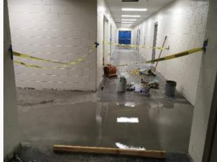
VCT Floor Leveling & Patch at Renovation
