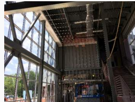
Lobby Window Wall, Duct, Ceiling Grid, & Gyp. Bd.
