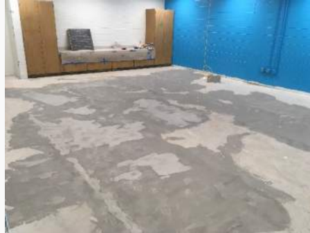
VCT Floor Prep & Moisture Remediation
