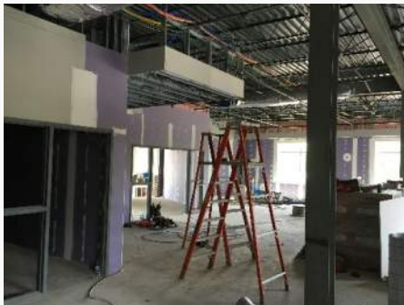
Media Center Soffits, MEP, & Gyp Bd.
