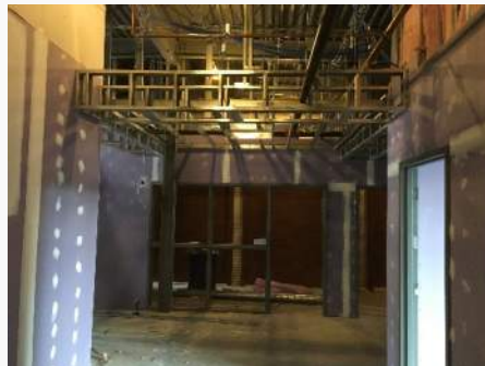
Hard Ceilings at New Building Restrooms & Corridors
