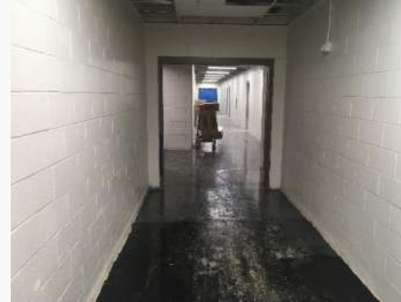
VCT Floor Prep & Moisture Remediation
