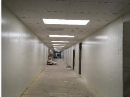
Ceiling Tile at Renovation
