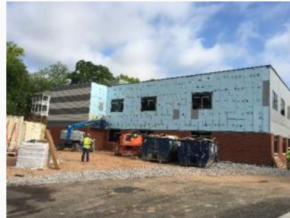
Window Frames/Glass & Metal Panels, & Insulation
