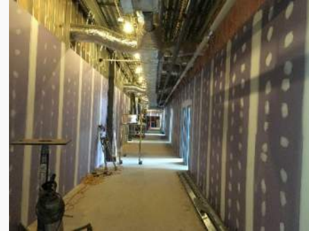
Two-Siding Gyp. Board Upper Level
