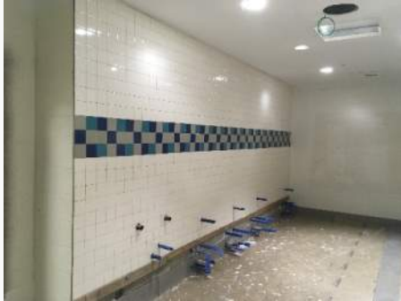
Wall Tile at Reno Restrooms
