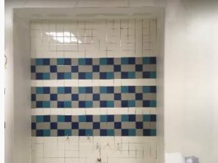
Wall Tile behind Water Fountains at Upper Level Addition
