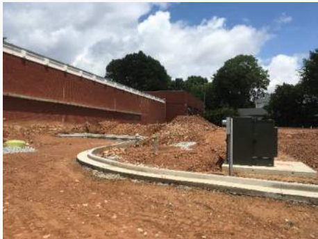
Curb and Gutter at Service Drive
