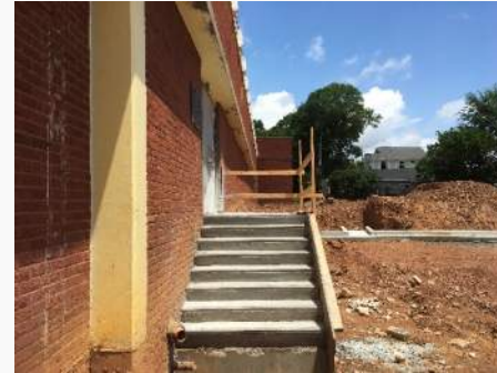
Ext. Conc. Stair at 60's Building
