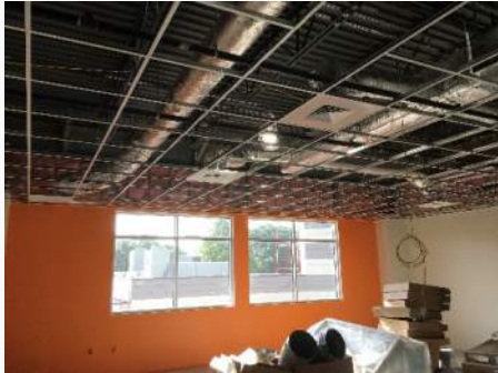
Paint & Ceiling Grid at Classrooms
