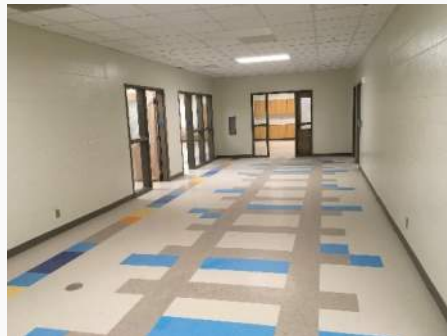
VCT Flooring at Reno Building Corridors
