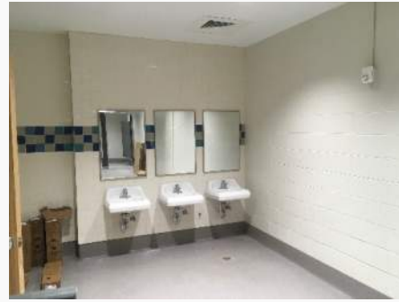
Bathroom Fixtures in Renovation
