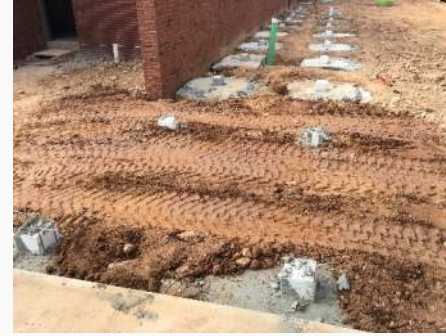
Canopy Footings at Courtyard
