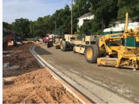
Curb & Gutter at Bus Loop
