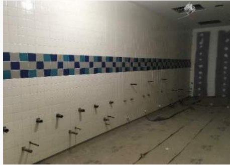
Wall Tile Bathroom Upper Level Addition
