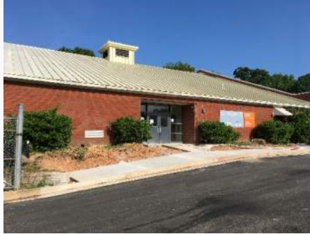
Sidewalks at Gym
