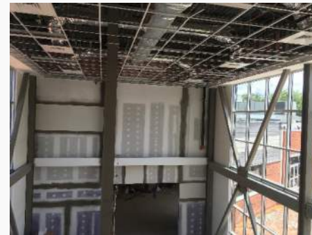
Lobby Window Wall, Duct, Ceiling Grid, & Prepped Gyp. Bd.
