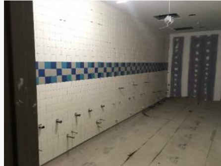
Wall Tile at New Building
