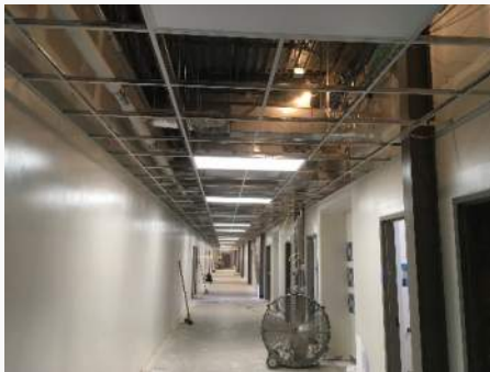
Ceiling Grid at New Building Upper Level
