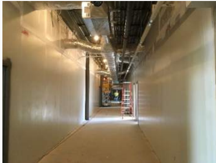
Painting Corridors at New Building Upper Level
