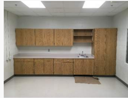
Millwork in Renovation
