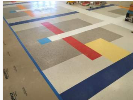
VCT Flooring at Auditorium in New Building
