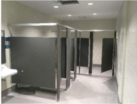
Bathroom Partitions in Renovation
