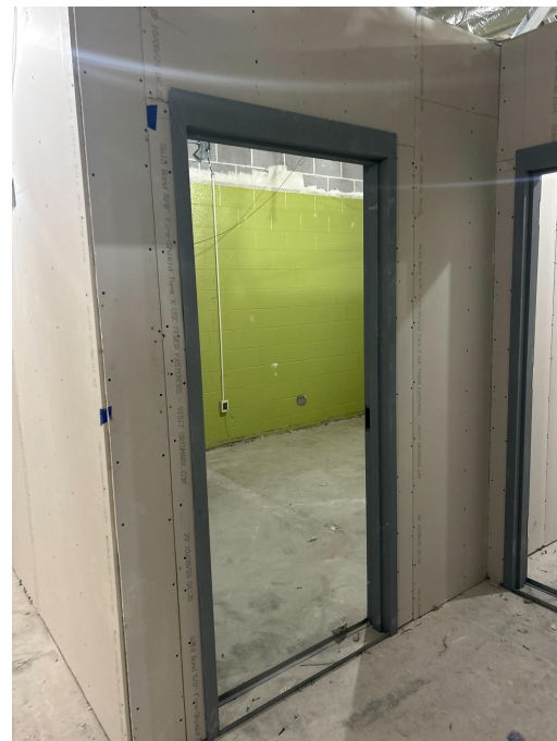
Setting door frames in classrooms on level 2.
