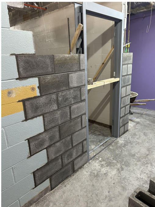
Setting door frames for masonry on level 2.
