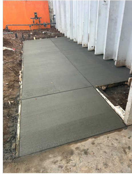
Concrete pads installed for mechanical units outside.
