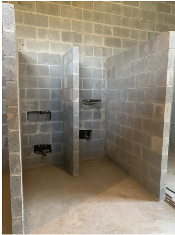
FD- Plumbing rough in
