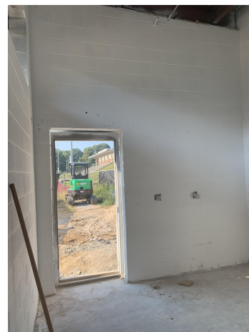
FD-Electrical rough in
