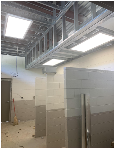
FD- Interior Light Install
