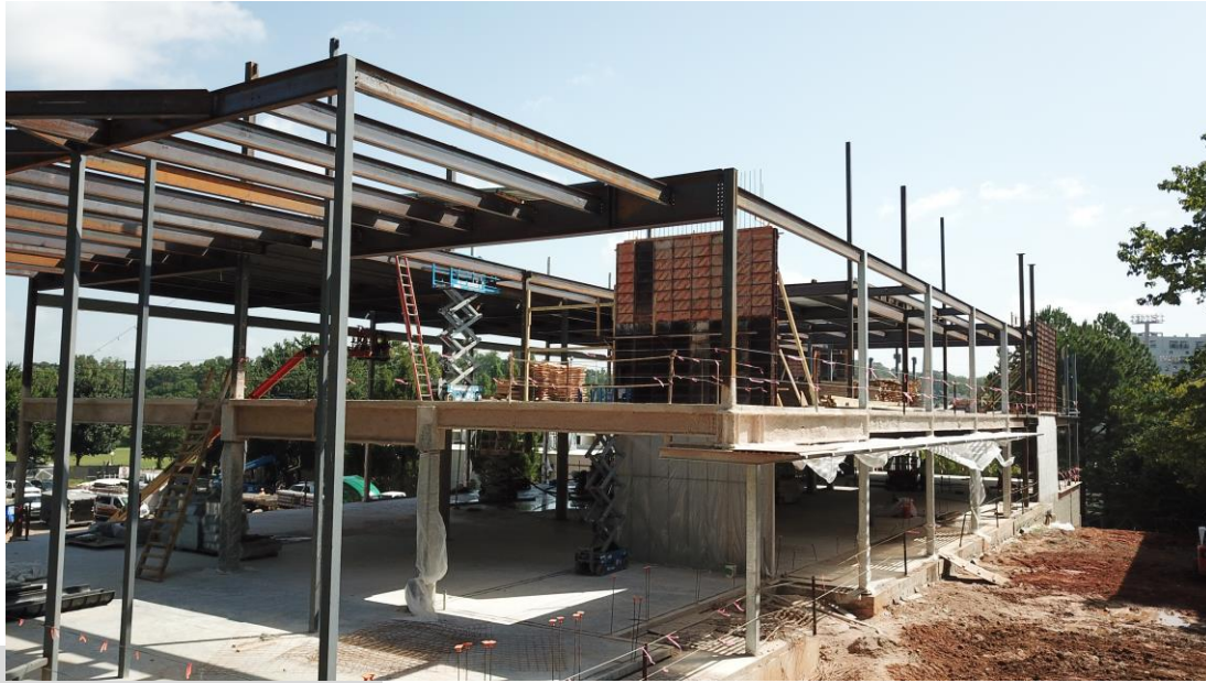
New Addition Progress
