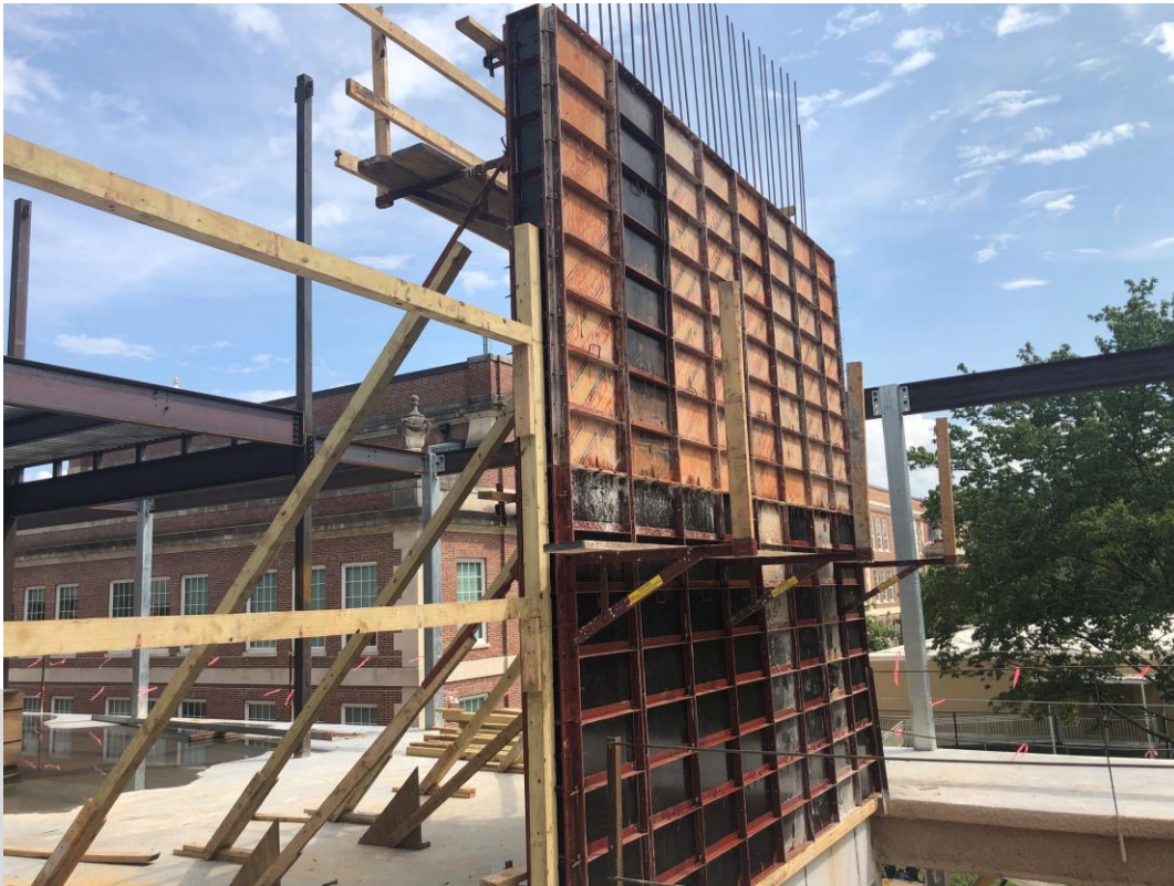
Forming Third Floor Shear Walls
