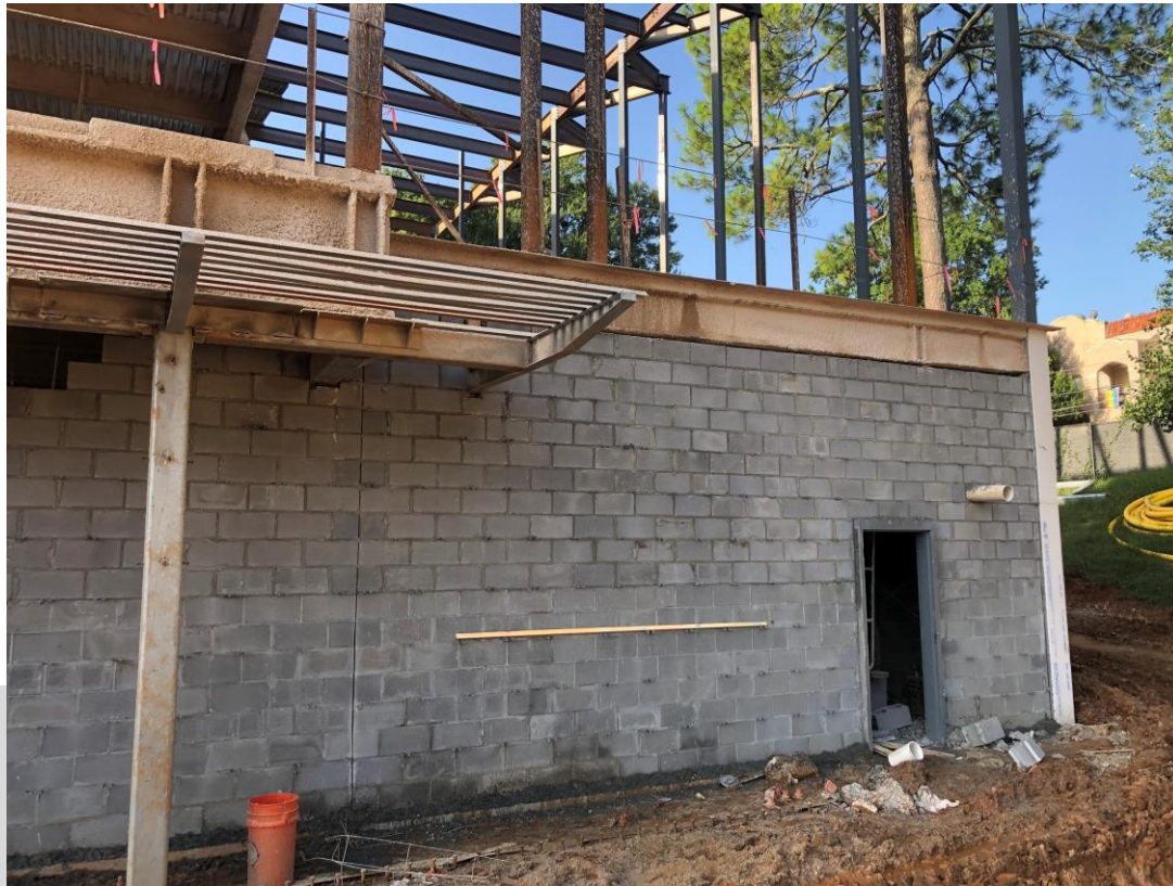
Northwest Exterior CMU Walls
