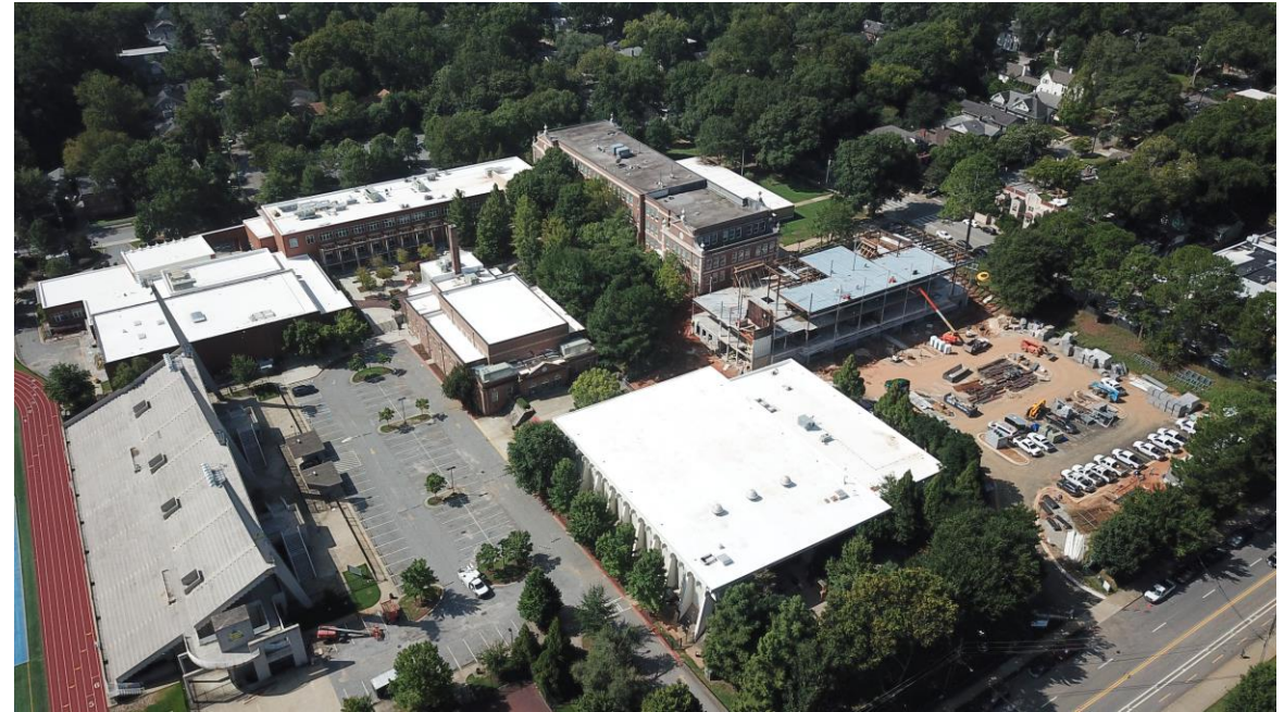
Overall Site Progress
