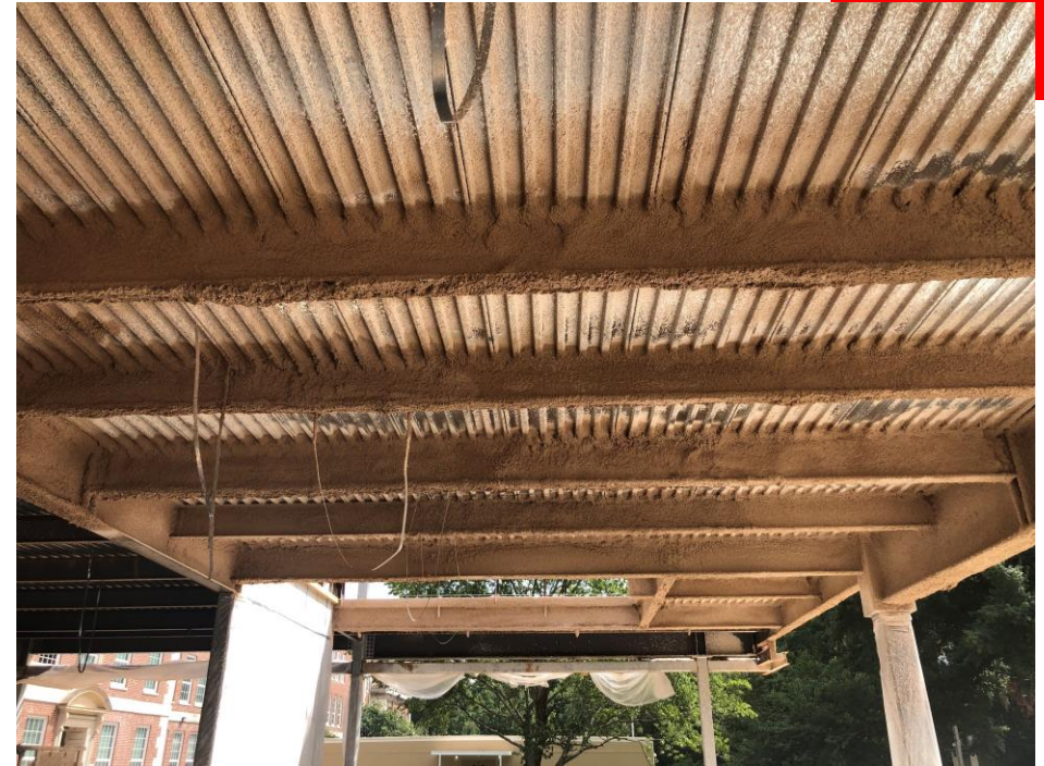
Second floor fireproofing
